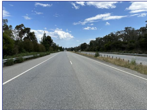
Figure 5: Western Port Highway - View South
