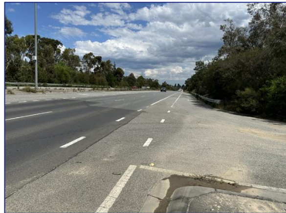
Figure 9: Intersection of Western Port Highway/Bellbird Court – View South
