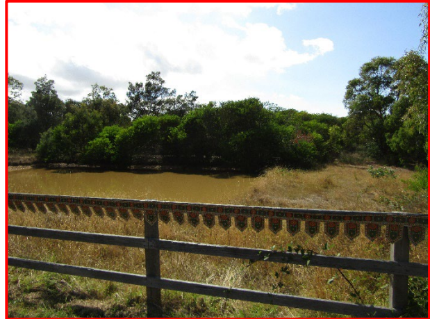
Plate 6 - View depicting the existing dam within the south east corner of the site
