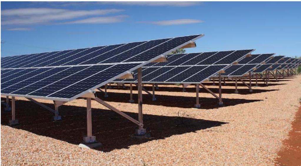
*Photo 1. Example of a typical fixed tilt system*
