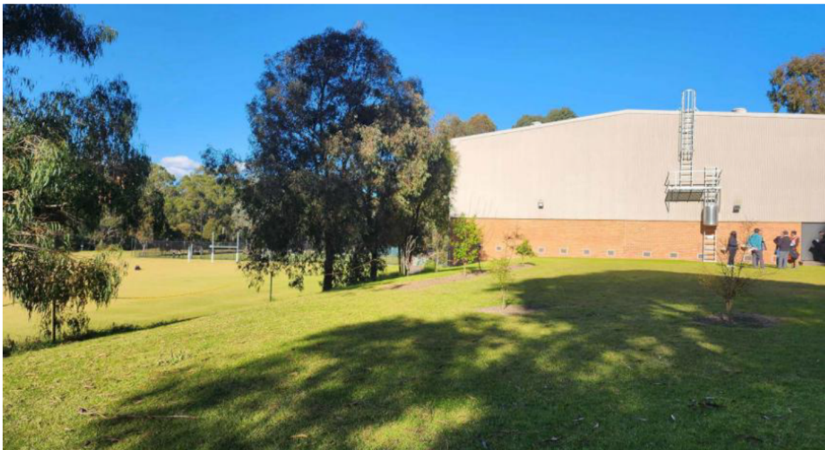
Figure 1 Existing gym as viewed from the north
