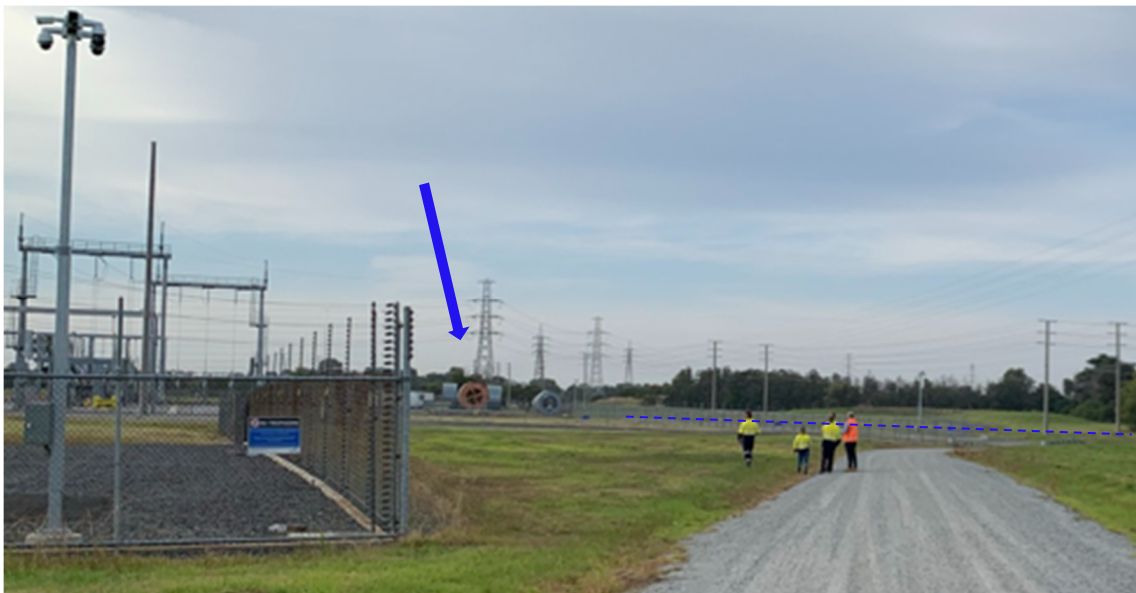
Figure 3: Ausnet Terminal Station looking south, approximate location of connection infrastructure and cable route
