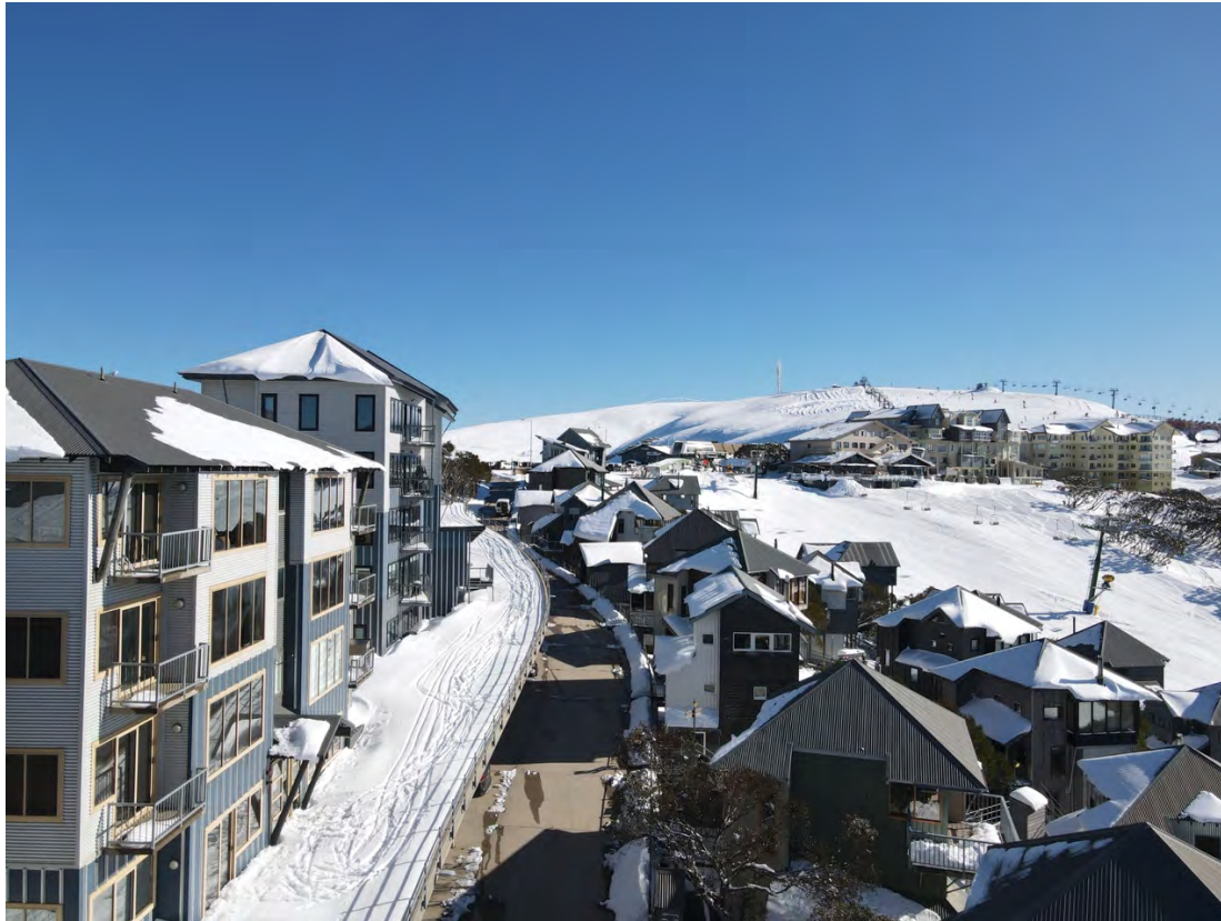
Hot Plate Drive looking north west
