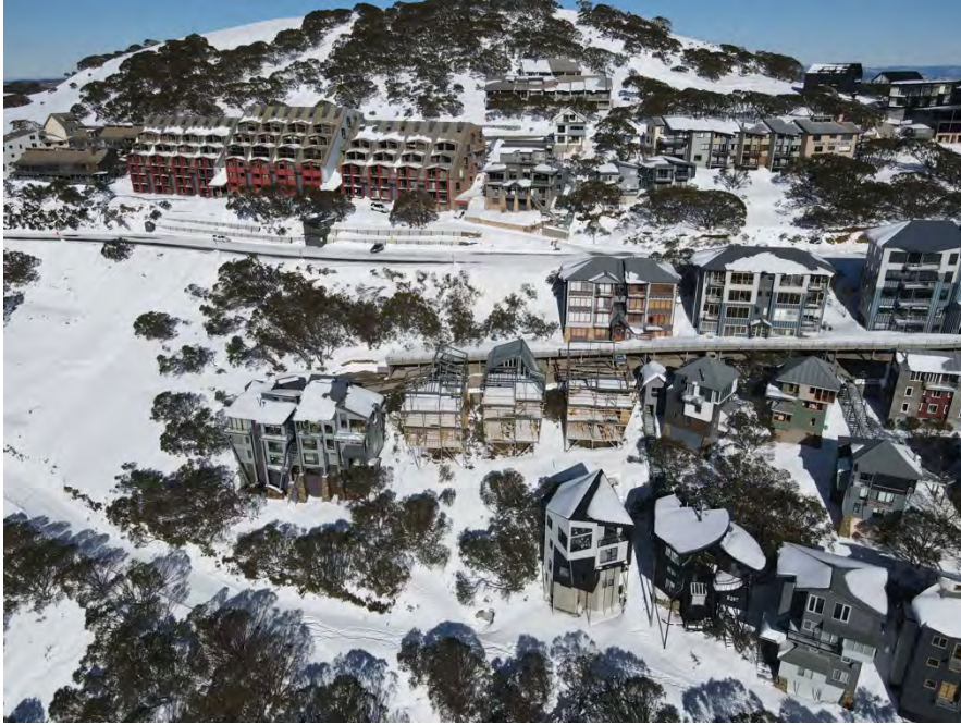
Figure 3.6: Subject land looking south west
