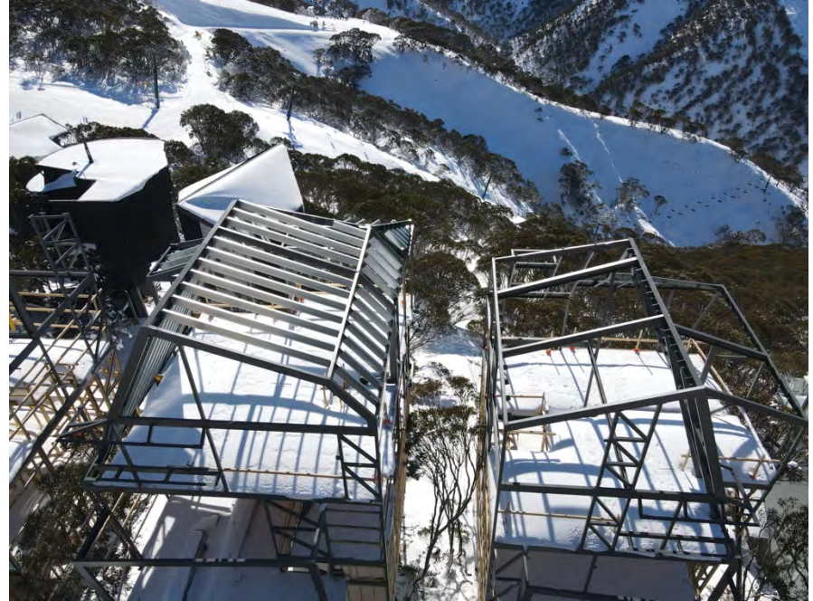
Figure 3.11: Overlooking from south abutting dwellings
