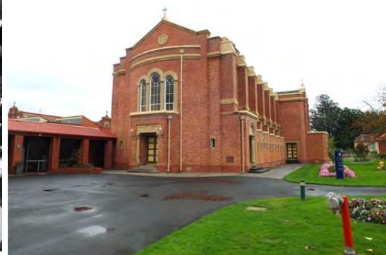
College Chapel, east and north elevations, 2014.
