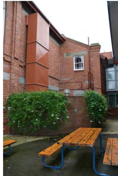
Healy Centre, south elevation (east end) showing original skillion lavatory wing, 2014.
