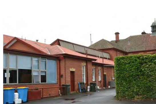
Kennedy House, south elevation (background), with kitchen in the middle ground and the flat-roofed dining room additions of 1961 in the foreground, 2014.
