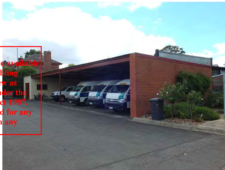
Former bus shelter/shed, west and south elevations, 2014.
