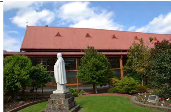
Whelan Food Centre (forming dining hall), west elevation (north end), March 2014.
