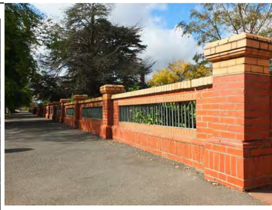
Front brick fence with altered central bays, 2014.
