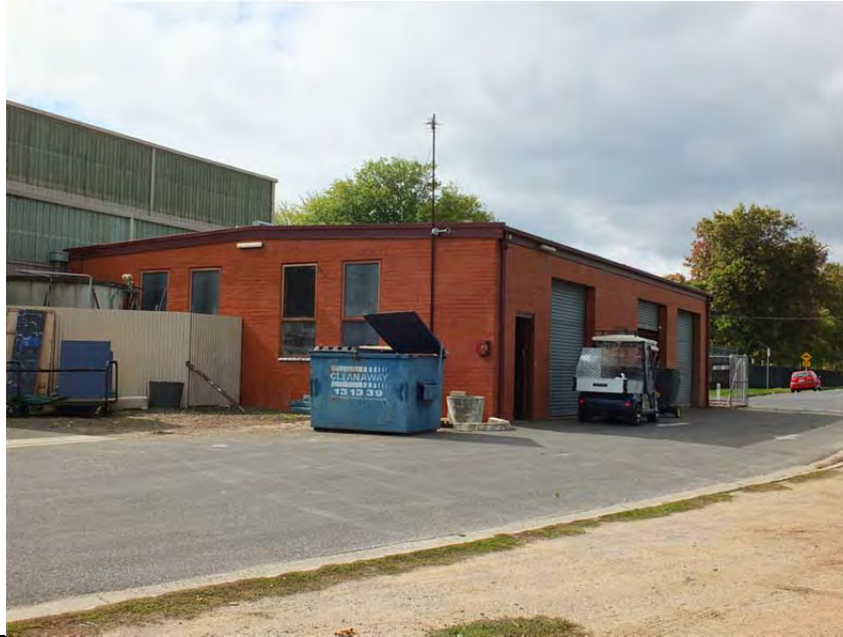
Maintenance Workshop, south and west elevations, 2014.
