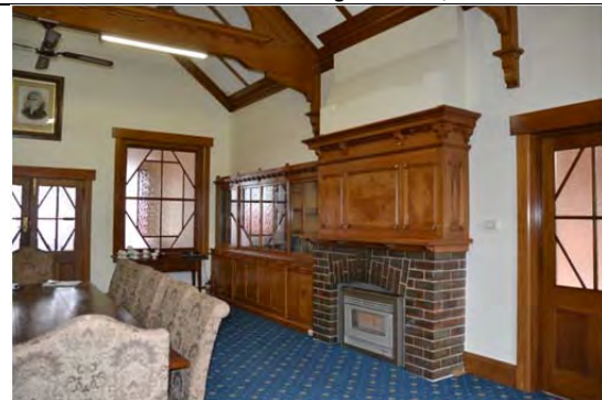
Former Library, Kennedy House, looking south-west showing fireplace and part of exposed timber trussed ceiling, 2014.
