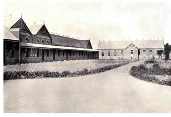
Library and Billiard Room addition (shown in the double gable ends on the left, brick classroom and the science wing on the right), 1916-17. Note post-support verandah that had been added in 1909. Source: St. Patrick's Annual, 1916-17.
