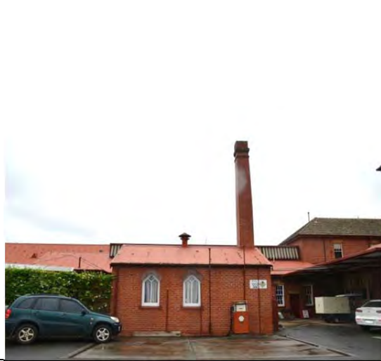
Kennedy House boiler room, east elevation, 2014.
