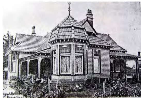
Nangle House (formerly 'Dimora'), front (north) and east elevations, 1906, prior to the verandah additions to the corner bay. Source: Ballarat Courier Christmas supplement, 5 December 1906, 1908 in Central Highlands Regional Library scrapbook collection, Ballarat.
