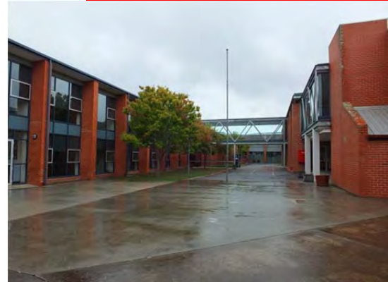
Kelty Court, looking west, 2014.
