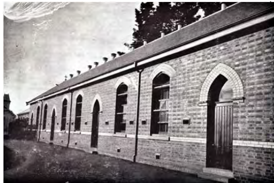
Brick Classroom (east wing – Pell Wing), west elevation, looking north, 1902. Note the absence of a verandah. Source: St. Patrick's College Annual, 1902.
