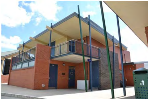
Kearney Stand, south and east elevations, 2014.
