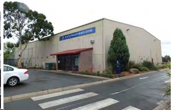
O'Malley Sports Centre, north and west elevations, 2014.
