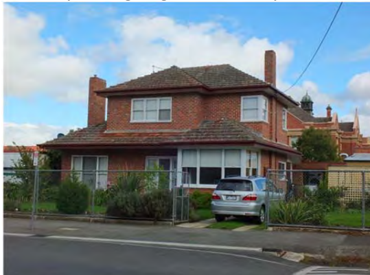
Wanliss House, front (east) elevation, 2014.
