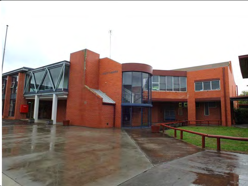
Edmund Rice Centre (former Kelty Centre), south elevation, 2014.
