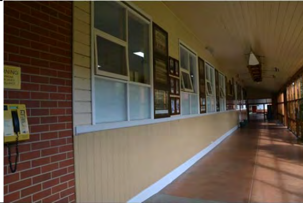
Whelan Food Centre (former dining hall), detail of west elevation under verandah, looking south, March 2014.
