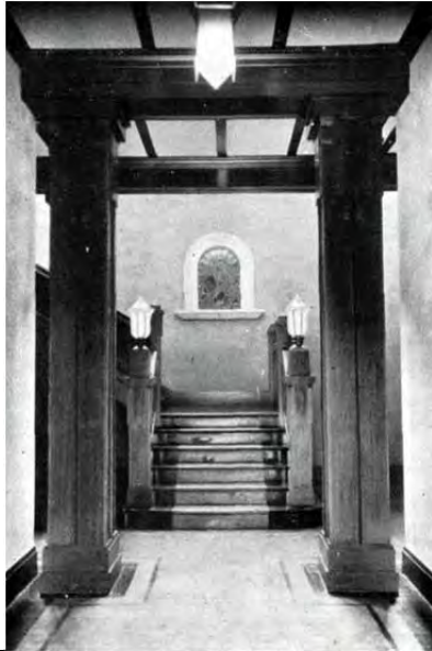
Kennedy House, entrance hall looking south to stair hall, 1933-34. Source: St. Patrick's College Annual , 1933-34.
