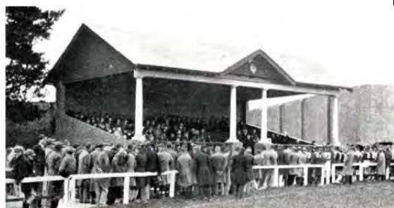
Opening day of Grandstand, 1932.
