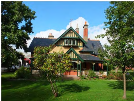
McCann House, north (front) elevation, 2014.
