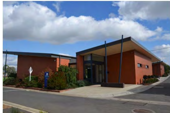
Old Collegians' Pavilion, east and north elevations, 2014.
