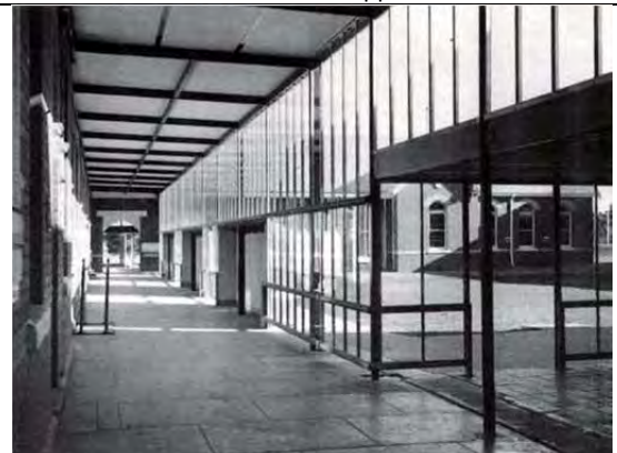
Interior view looking south (classroom wing on left and old Science Wing in background on right), 1977, showing recently completed glazed in verandahs. Source: St. Patrick's College Annual, 1977.
