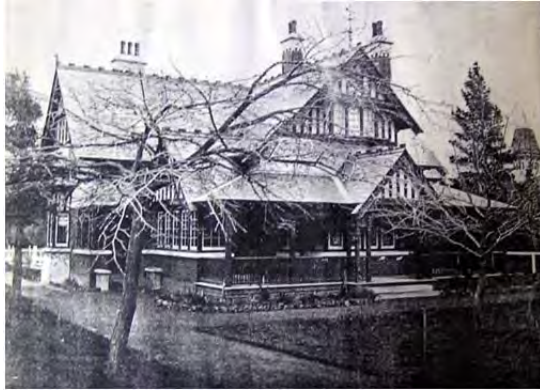
McCann House (formerly 'Dallata'), 1908. Source: The Courier Christmas supplement, 15 December 1908 in Central Highlands Regional Library scrapbook collection, Ballarat.
