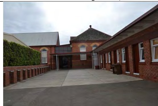
Pell Wing, south elevation (science wing to the left and the south addition to the brick classroom to the right), March 2014.
