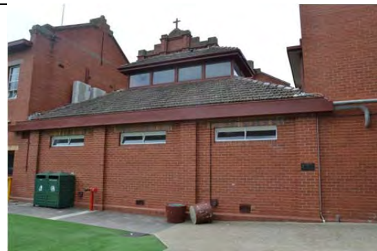
Purton Centre – detail of shower wing, west elevation, March 2014.
