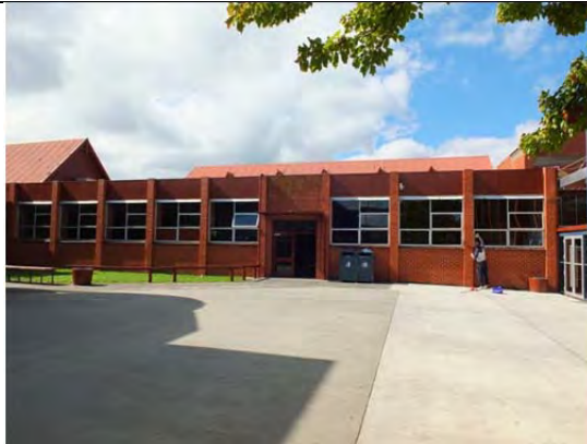
Heinze Theatre showing west elevation of Assembly Hall, 2014.
