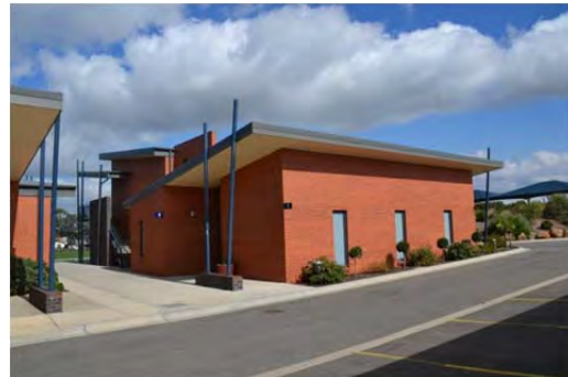
Kearney Stand, east and north elevations, 2014.
