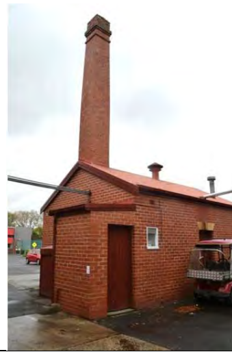
Kennedy House, boiler room, north and west elevations, 2014.
