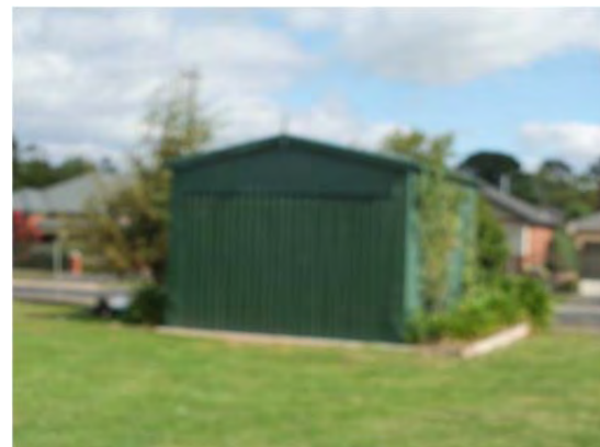
Shed to west of Hill Oval, east and north elevations, 2014.
