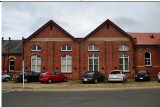
East elevation of former library and billiard room, March 2014.
