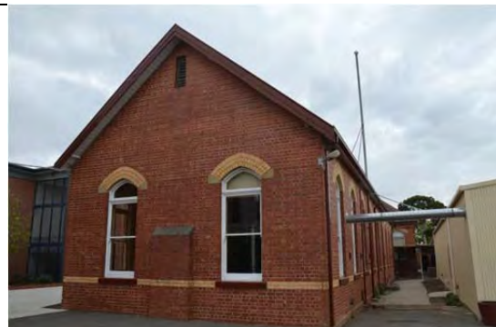
Pell Wing (old Science Wing), west elevation, March 2014.
