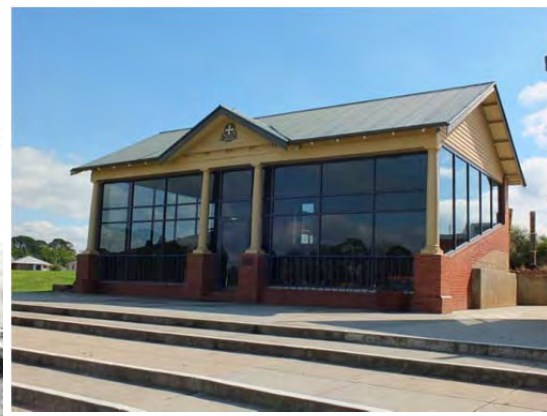
Stewart Theatre, south and west elevations, 2014.
