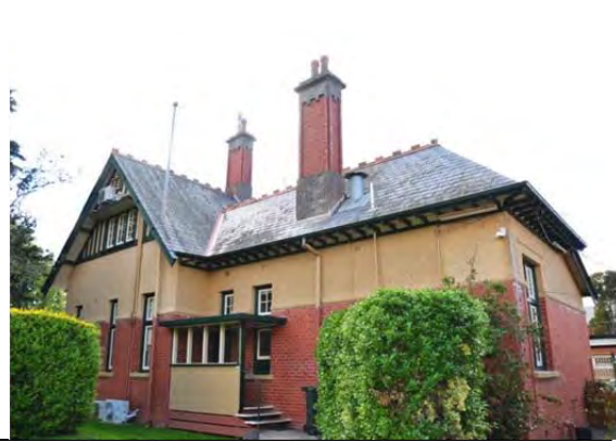
McCann House, west elevation, 2014.
