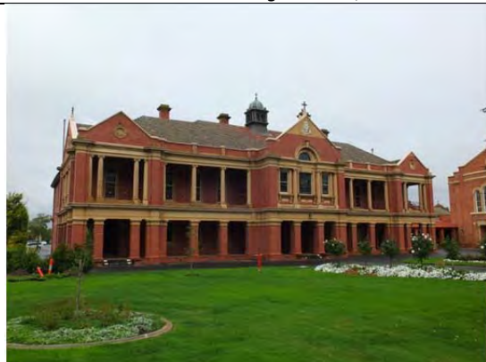
Kennedy House, north elevation, 2014.
