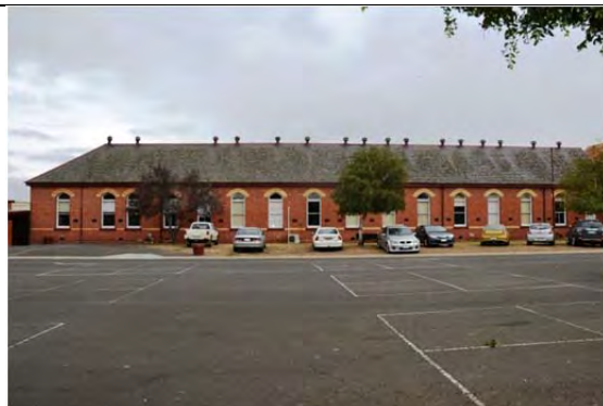
Pell Wing (early brick classroom), east elevation, March 2014.
