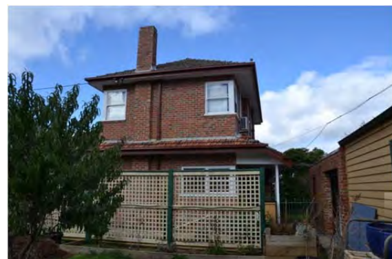
Wanliss House, north elevation showing rear early brick outbuilding, 2014.
