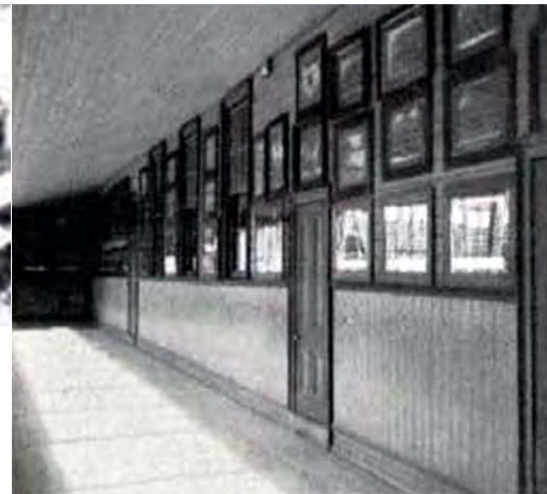
Whelan Food Centre (Dining Hall), showing west elevation under verandah, 1941-42. Source: St. Patrick's Annual, 1941-42.
