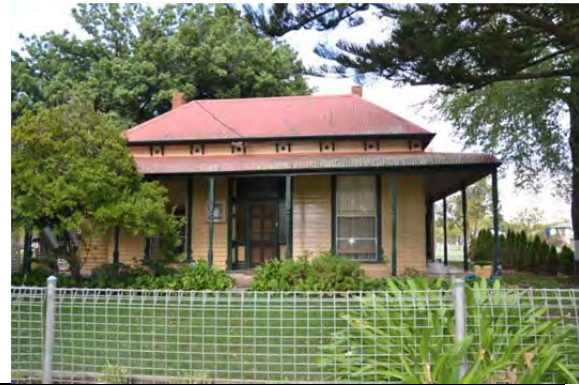
McCunnie House, front elevation with front fence, 2014.
