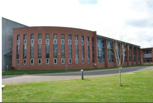
Wilding Wing, rear (south) wing, west and south elevations, 2014.
