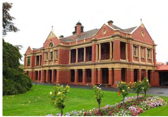
Kennedy House, north and west elevations, 2014.
