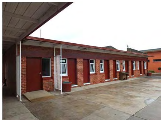
Change Rooms, west elevation, 2014.
