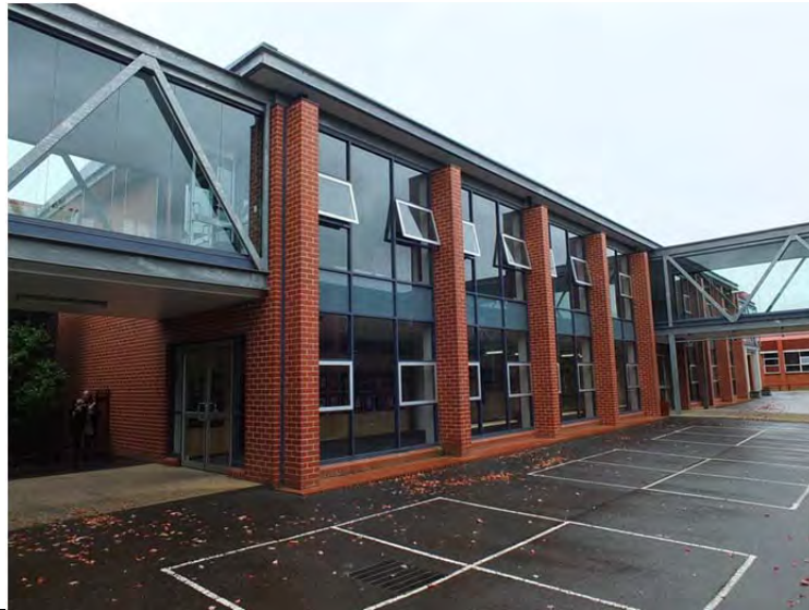
Little Wing, south and west elevations, 2014.
