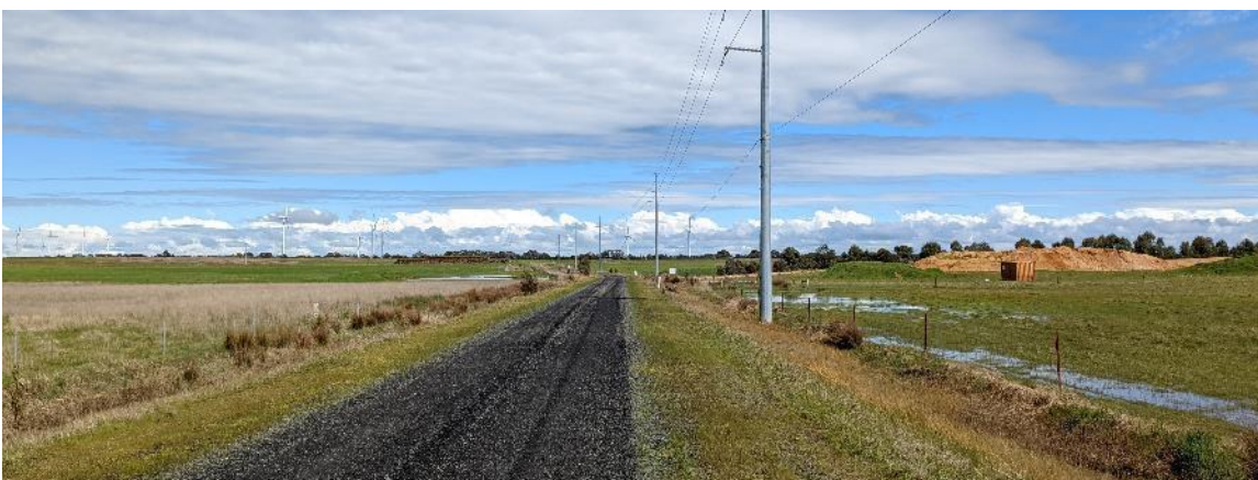
Figure 10 – Unnamed access road adjacent to the site looking west
