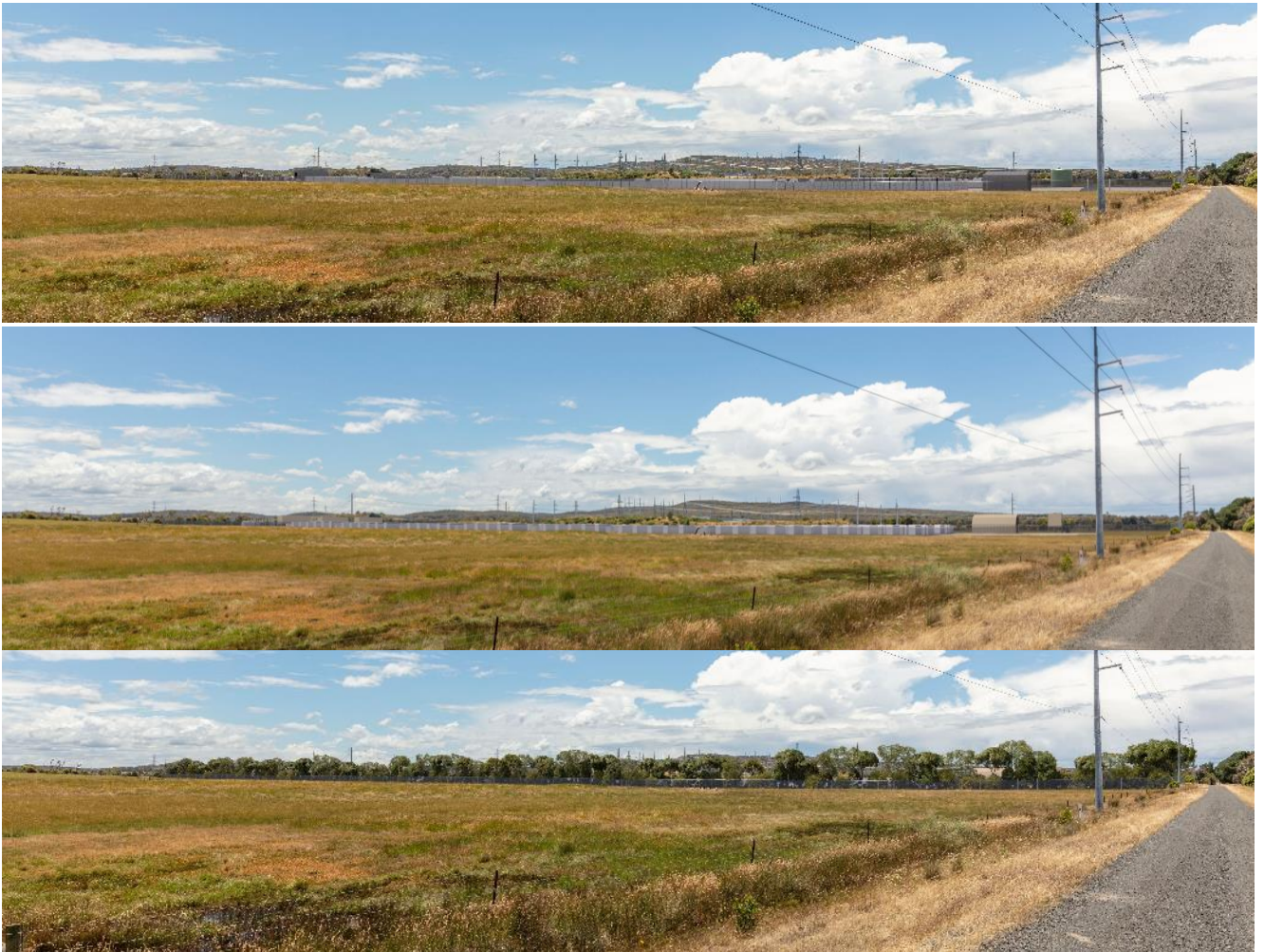
Figure 25 – Elaine BESS from Position 01 – permit plans proposed built form (top), proposed amendment built form (middle) and with native vegetation screening (bottom)
