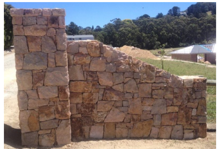
Stone entry wall and signage credit: basysidestoneconstruction.com.au Non combustible
