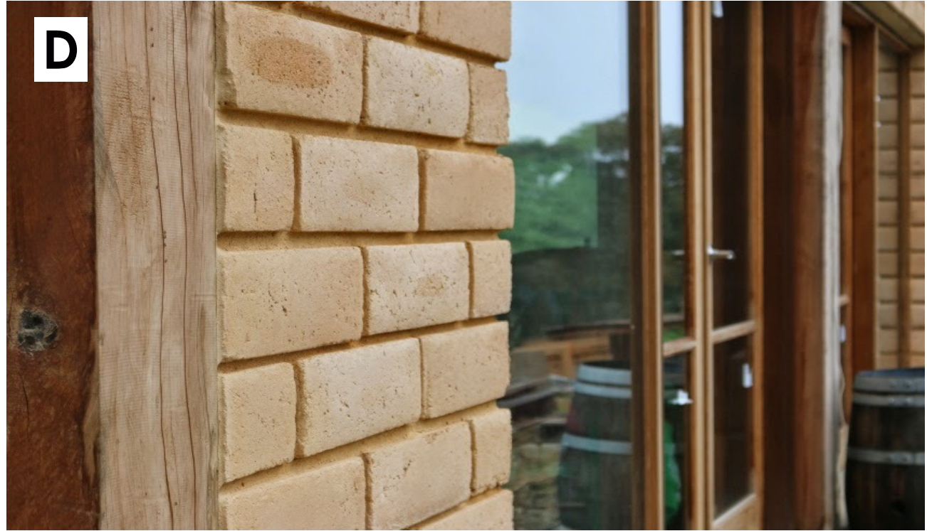
Timbercrete block external walls and timber feature entry doors credit: timbercrete.com.au BAL 29 or higher
