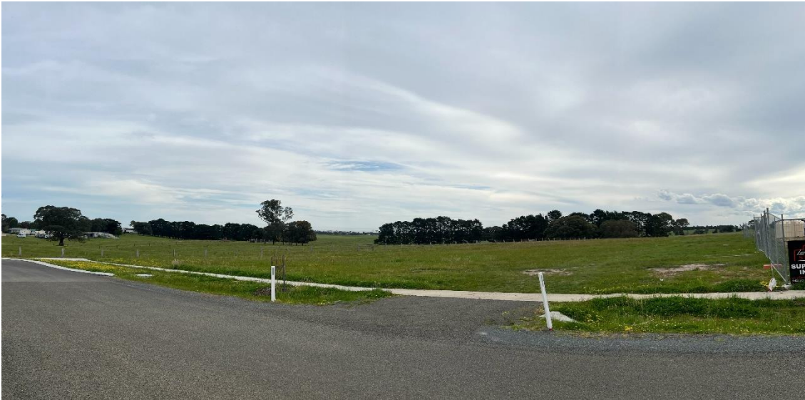
Frontage to Caldwell Court looking west, showing transition from kerb and channel to swale drainage
