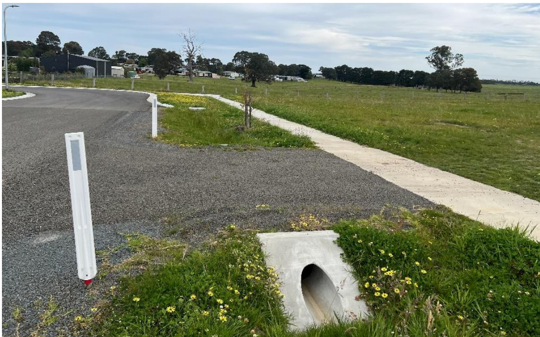
Frontage to Caldwell Court looking south, showing transition from kerb and channel to swale drainage
