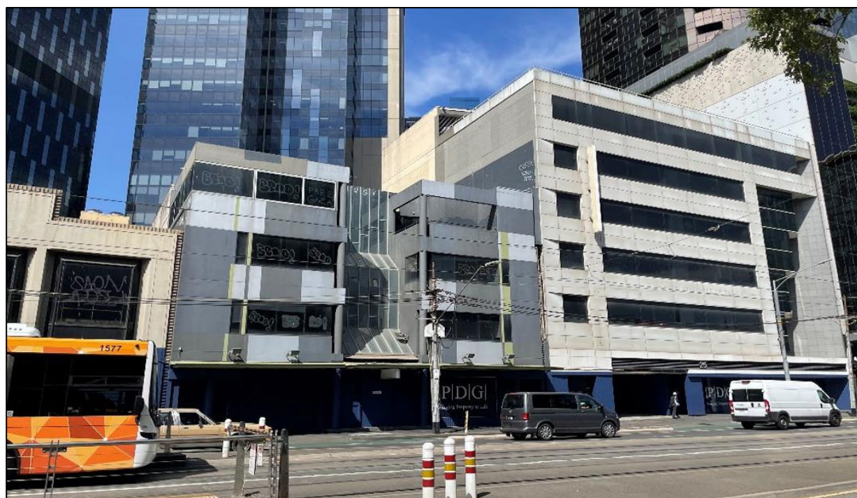
Figure 15: 17-23 and 25-29 Queens Bridge Street (Source: Application)
