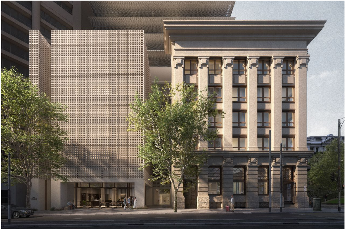
Figure 38 View from Collins Street showing the effect of the deeply recessed transitional floor levels Source: Carr Architects
