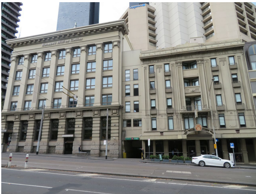
Figure 22 The former State Savings Bank to the left, adjoining the subject site via the later infill between the two buildings
