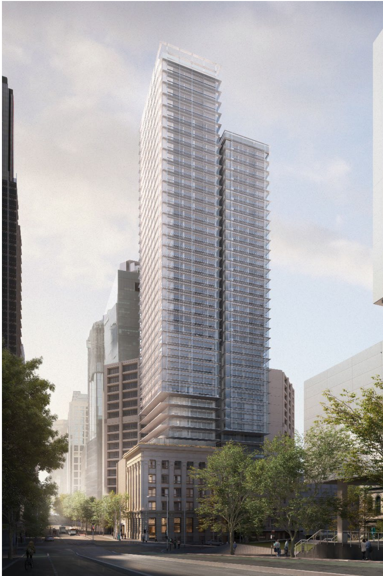
Figure 40 Longer view from the south along Spencer Street Source: Carr Architects
