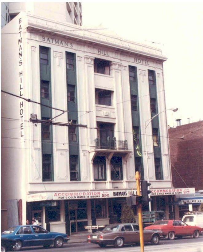
Figure 13 Image of the Batman's Hill Hotel included in the 1985 Building Identification Form. Note that the rendered brick dados were still partially intact at this point. Source: Graeme Butler via Hermes Database, Department of Environment, Land, Water and Planning
