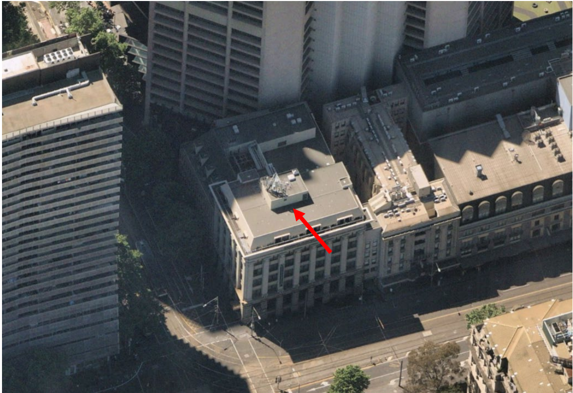
Figure 33 Later mansard roof and sixth floor level to be removed indicated by the red arrow Source: Nearmap October 2021
