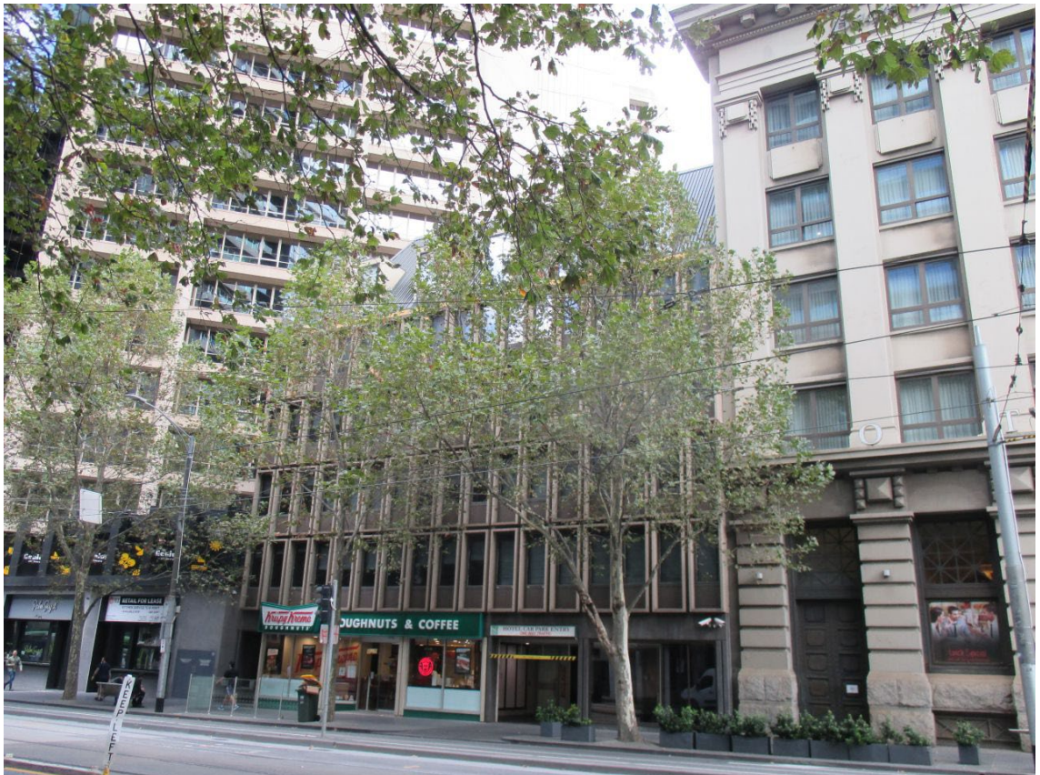
Figure 25 The modern infill building at 607-613 Collins Street from Collins Street
