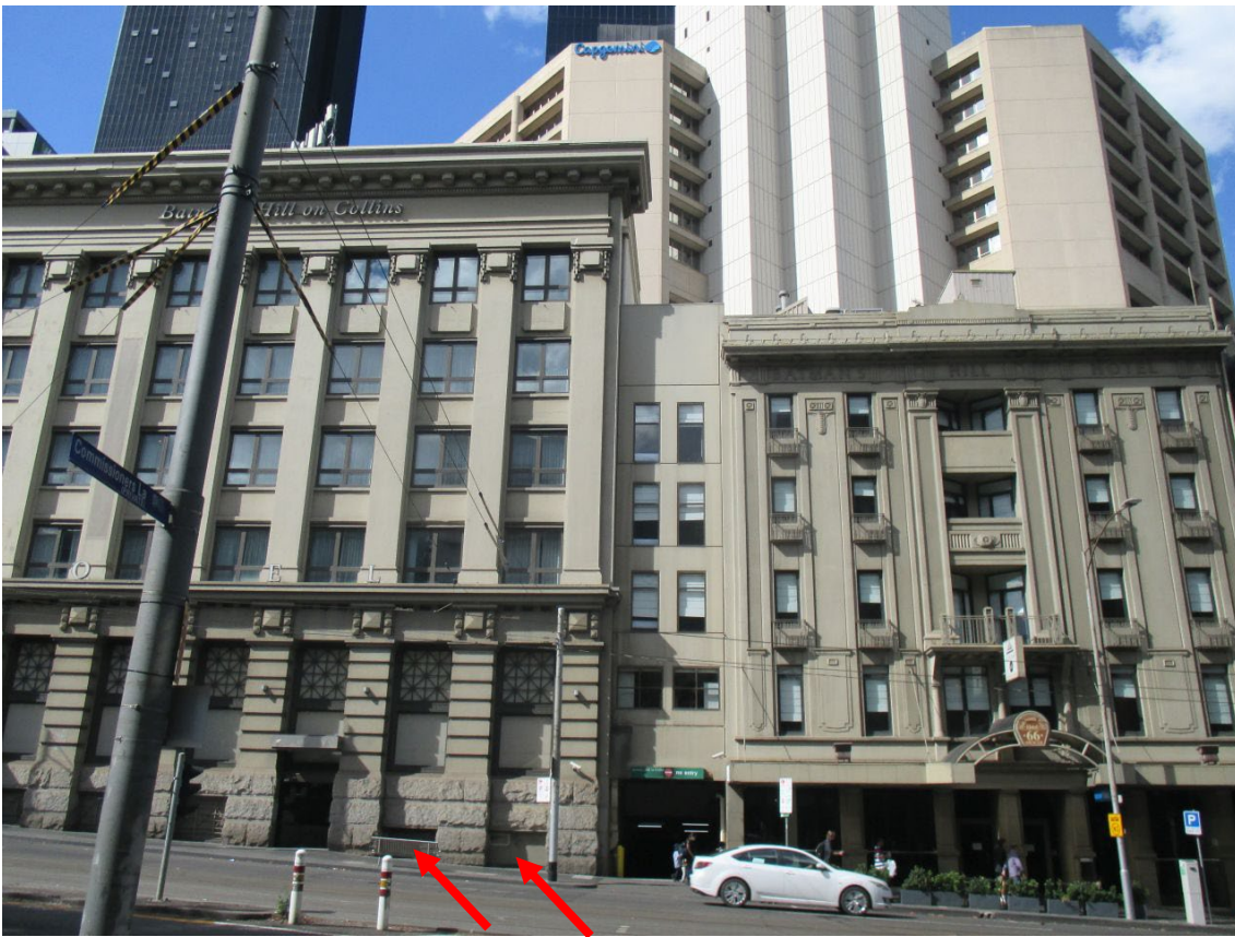
Figure 30 Location of granite to be removed indicated by the red arrows
