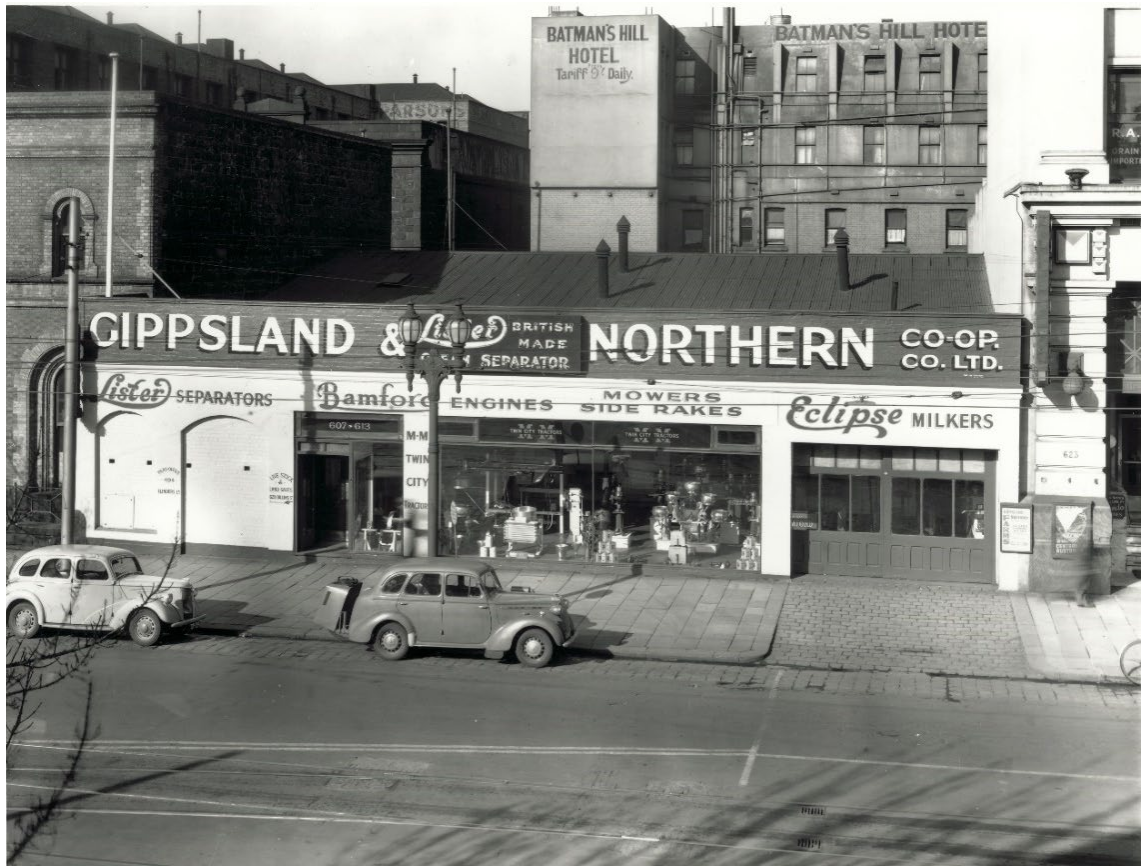
Figure 8 The earlier building at 607-613 Collins Street, c. 1940. Note the north elevation of the Batman's Hill Hotel in the background Source: H.H Paynting, SLV file pi009814
