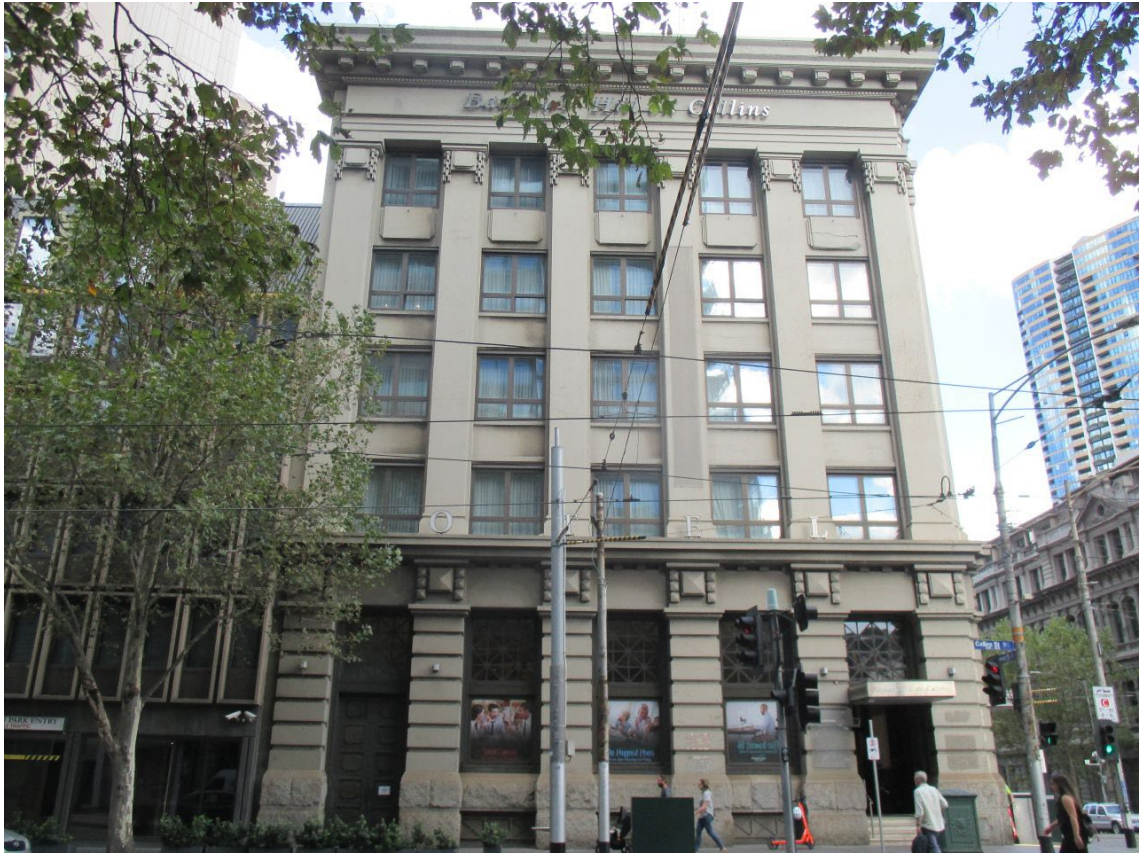
Figure 18 The State Savings Bank façade from Collins Street
