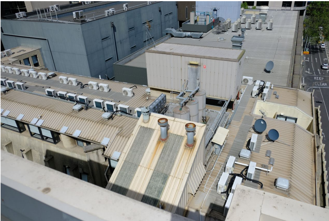
Figure 34 The roof of the Batman's Hill Hotel showing the modern mansard roof to the added fifth level.
