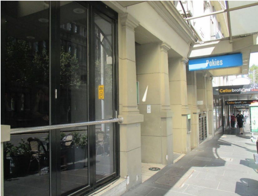
Figure 36 Later alterations to the street level Collins Street elevation including enlarged openings, inset door, modern windows and doors, glazed arched awning and re-rendered façade
