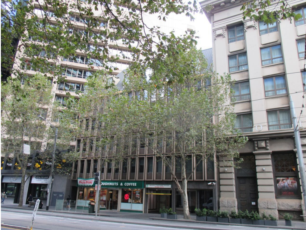
Figure 2 The modern infill building at 607-613 Collins Street from Collins Street
