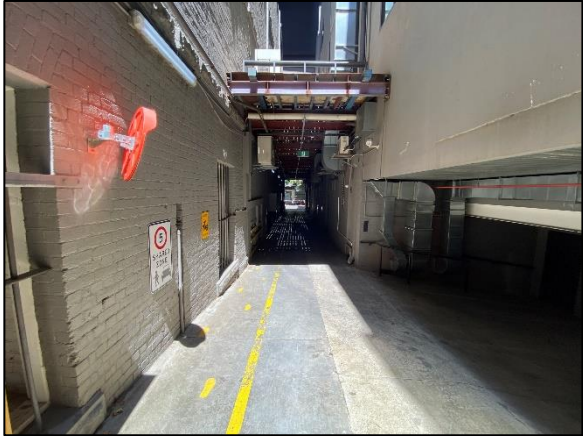
Figure 13: Private Laneway - View South
