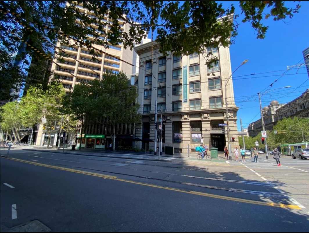
Figure 3: Site Frontage - View from Collins Street
