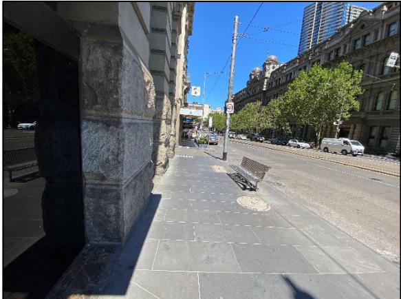
Figure 17: Spencer Street Frontage - View South
