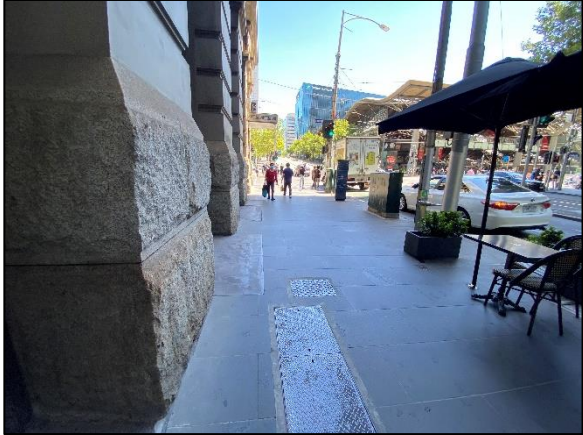
Figure 15: Collins Street Frontage - View West
