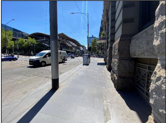
Figure 16: Spencer Street Frontage - View North
