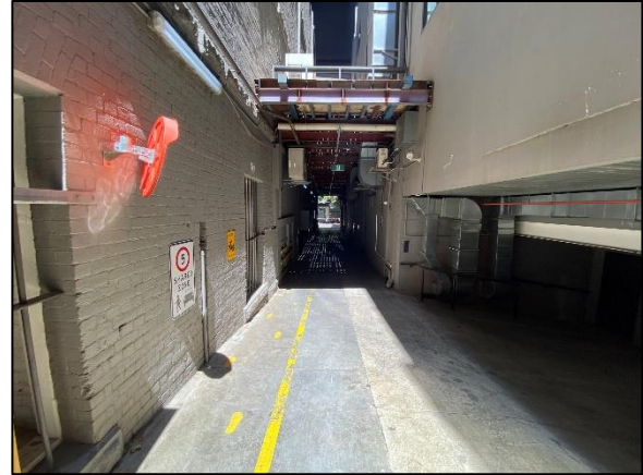
Figure 13: Private Laneway - View South
