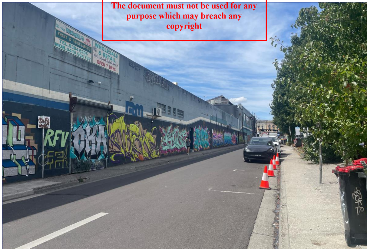
Figure 6: Subject Site – view north-east from Florence Street
