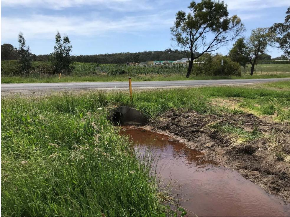
Photo 1 – External catchment flows received from the culvert beneath Horswood Road, north-east of the site.
