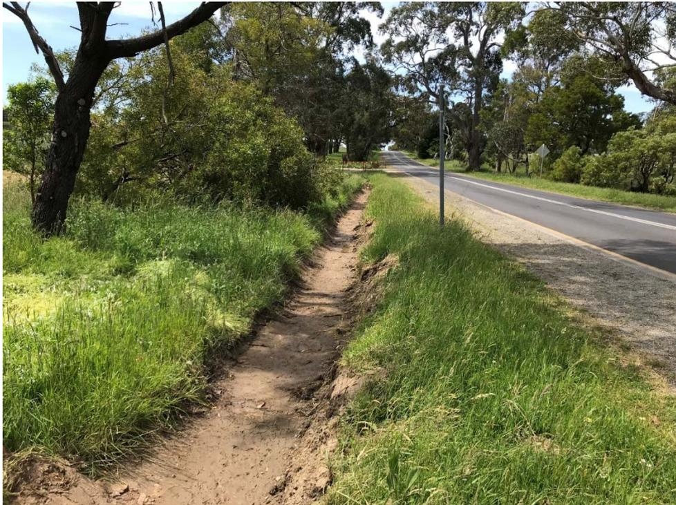
Photo 3 - External catchment open drain north-east of the site, on north side of Horswood Road.
