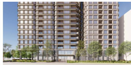
Figure 15: View from St Kilda Rd
