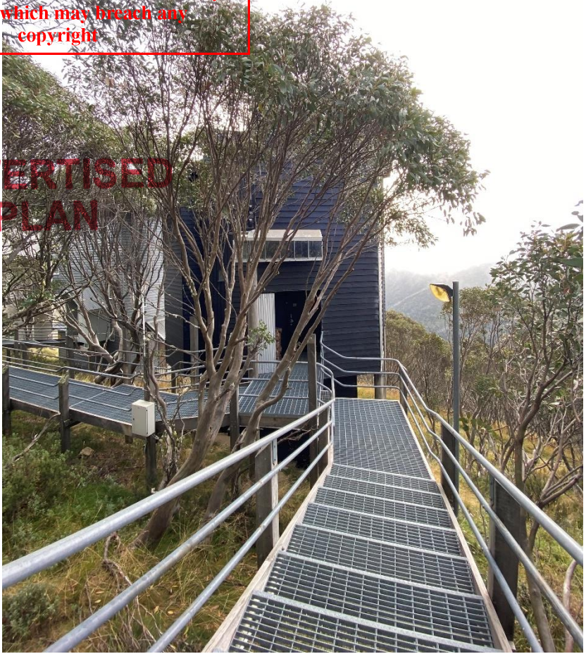
Common stairway alongside Lot 31 looking at Lot 32
