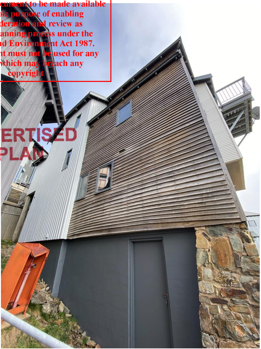
Existing building on Lot 20 with windows overlooking Lot 22
