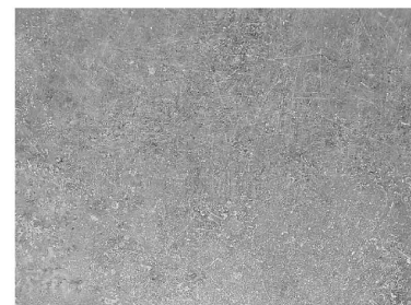
CO: DRIVEWAY CONCRETE
