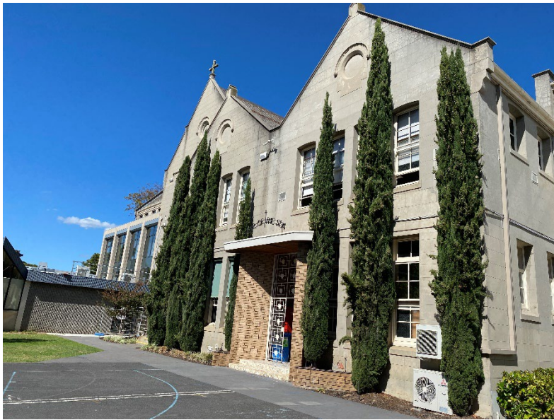
Figure 6. View from the northwest of Trees 68-70 Cupressus sempervirens 'Stricta' in their growing environment. (Ido Monk, April 2022).
