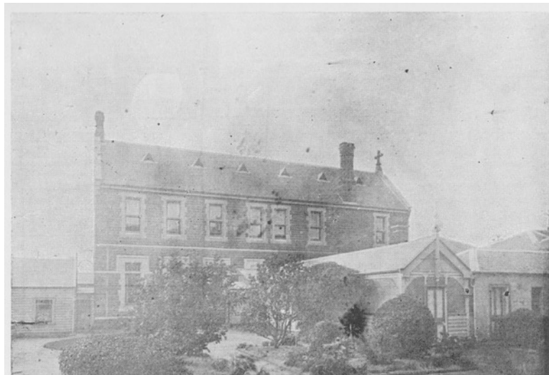
Figure 4: Photograph of the first stage of the Heritage Wing, completed in 1886, viewed from the south. (Source: Some of the Fruits of Fifty Years).
