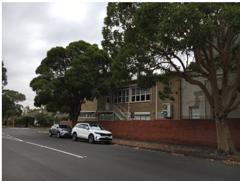
Figure 14: Science Block built 1966, adjacent to the corner of Martin and Murphy Streets (viewed from Murphy Street). It is proposed to be removed as part of the works for the STAR Centre.
