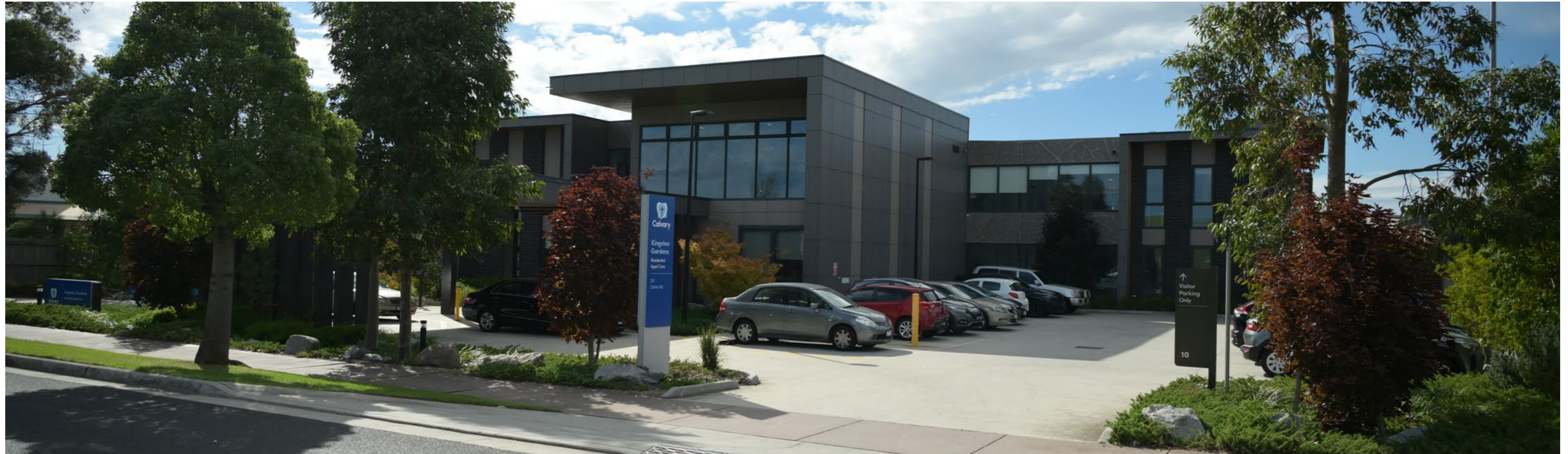
Figure 6-6 Existing Landscaping within the frontage of the aged care facility.
