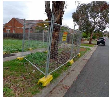
Figure 3: Tree protection fencing around a single tree in a nature strip setting.
