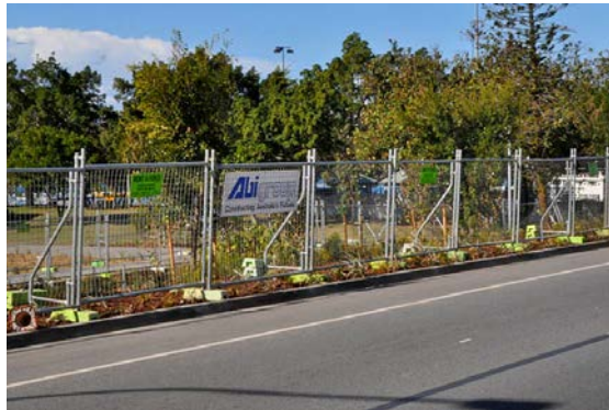
Figure 2: Tree protection fencing across a long section
