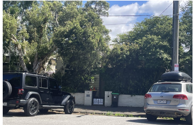
Figure 20 – The single storey residence at 14 Grosvenor Street.
