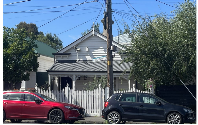
Figure 30 – The single storey Victorian at 11 Brunning Street.
