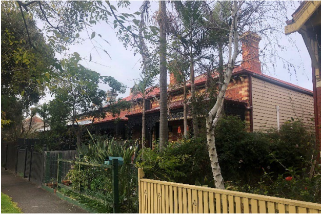
Figure 23 – The polychrome brick Victorian at 21-25 Grosvenor Street.
