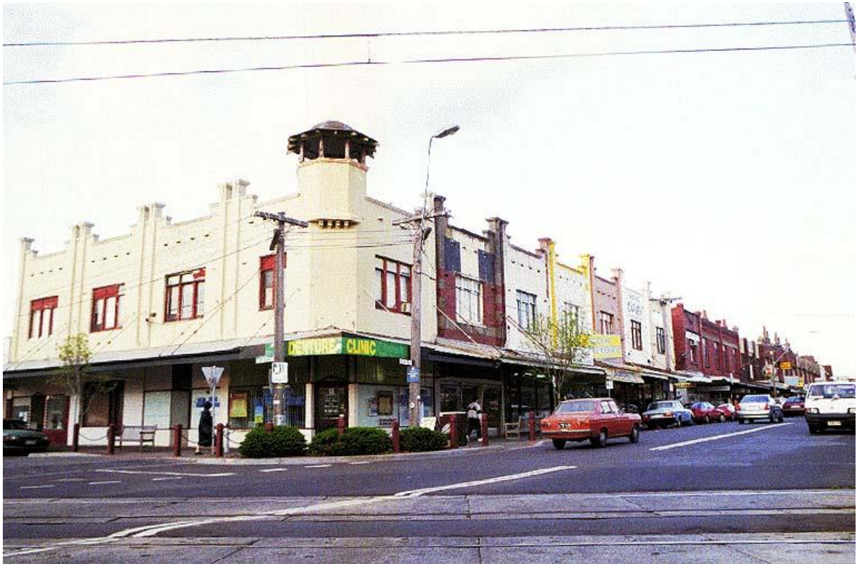
Figure 6.11-10 – The Glen Eira Road centre commences at the railway line with this group of shops erected in 1912. Though transformed by the present coat of paint, the façade treatment is representative of the centre yet enhanced by the corner tower.
