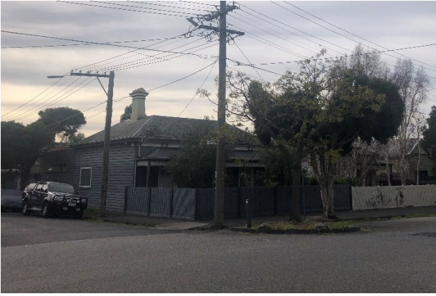
Figure 17 – The single storey Victorian dwelling at 10 Grosvenor Street.
