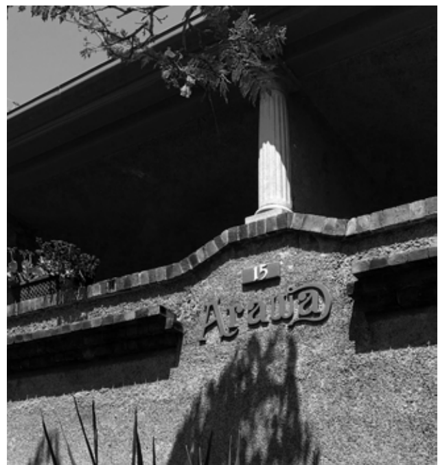
Photo 4. This block of flats in Wimbledon Avenue retains original finishes including the clinker brickwork, which contrasts with the natural (unpainted) render.
