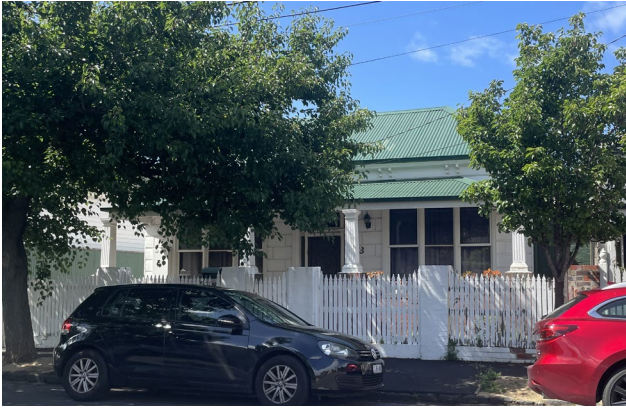
Figure 29 – The single storey Victorian at 13 Brunning Street.
