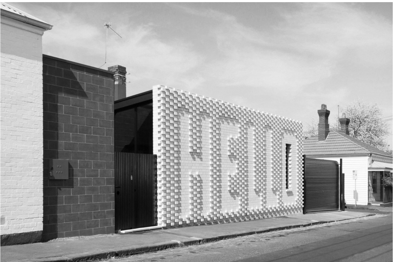
Photo 11. An extension featuring Hello wall by architect Fook-Ling Khoo and graphic artist Rose Nolan. This design elevates a practical solution for privacy by creating "Hello" out of fine brickwork. It also showcases how contemporary design can contribute to the brick tradition of its 19th century heritage neighbours.
