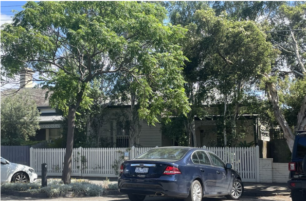
Figure 19 – The single storey residence at 12 Grosvenor Street.
