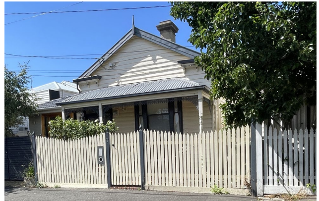
Figure 32 – The paired timber Victorian buildings at 5-7 Brunning Street.
