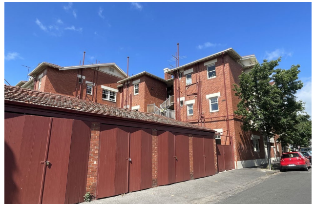
Figure 34 – Rear of the Yurunga apartments and single storey garages to 36 Brighton Road.
