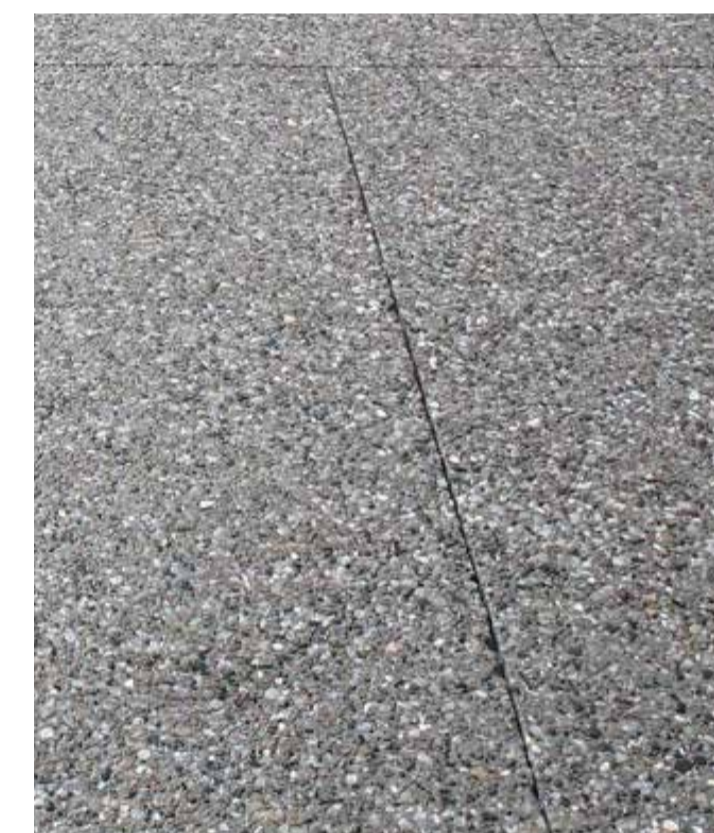
Exposed aggregate coloured concrete paving (green Envirocrete) supplied by Boral
