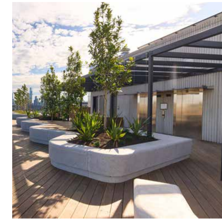
Smaller planters may include off white GRC over basement areas
