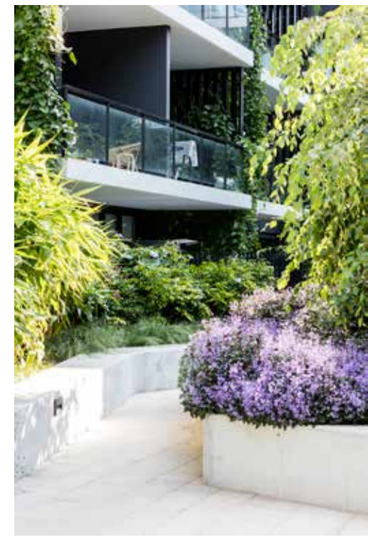
Off white institute raised planters over basement areas providing a seating edge typically 500mm above FSL
