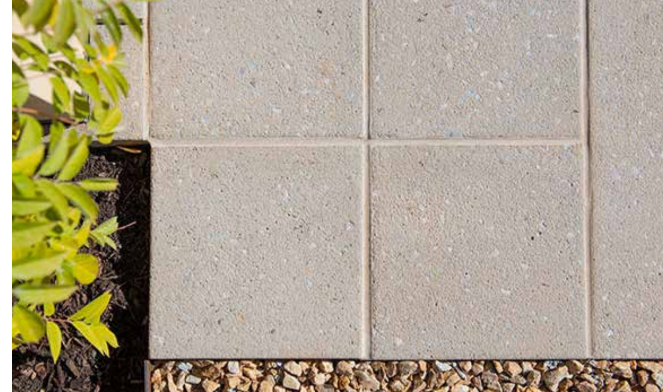
Precast concrete square pavers laid over concrete slab
