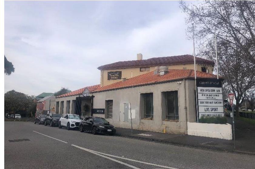
Picture 4 – Rear of Grosvenor Hotel (along Grosvenor St)
