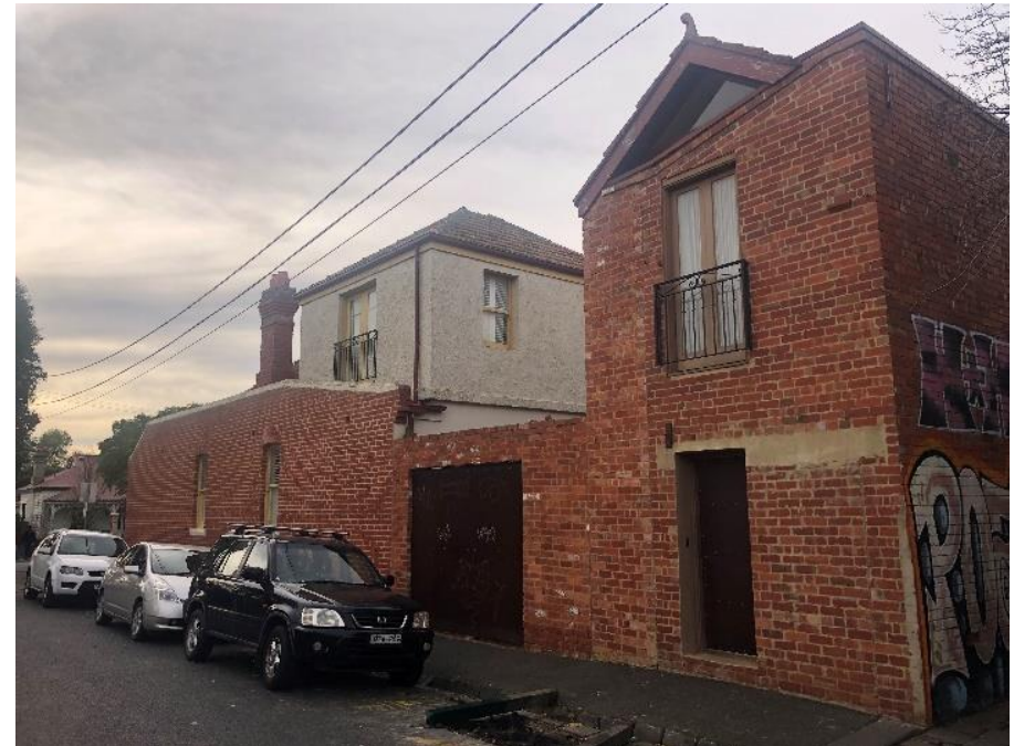
Picture 2 – Existing built form on east side of Woodstock St (rear of 19 Grosvenor St)
