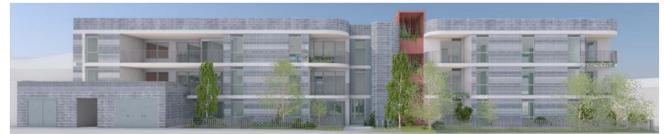
Figure 5 – Brunning St elevation, showing stairwell / main entry articulation.
