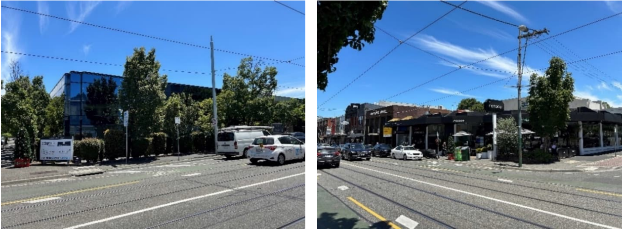
Figure 9: Photographs of No's 797-799 and 801-805 Glenferrie Road
