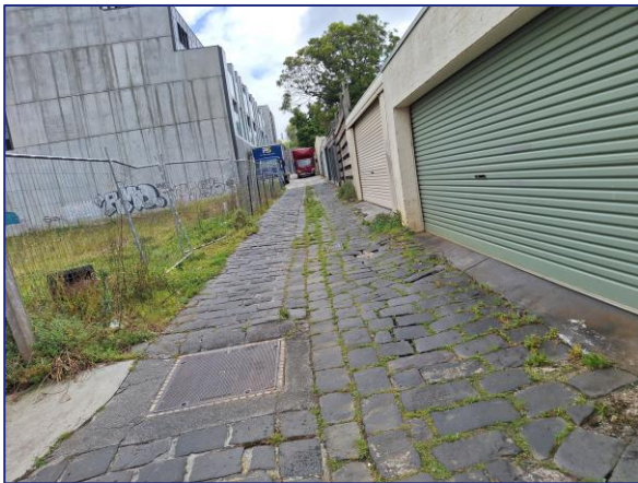
Figure 9: ROW – view north
