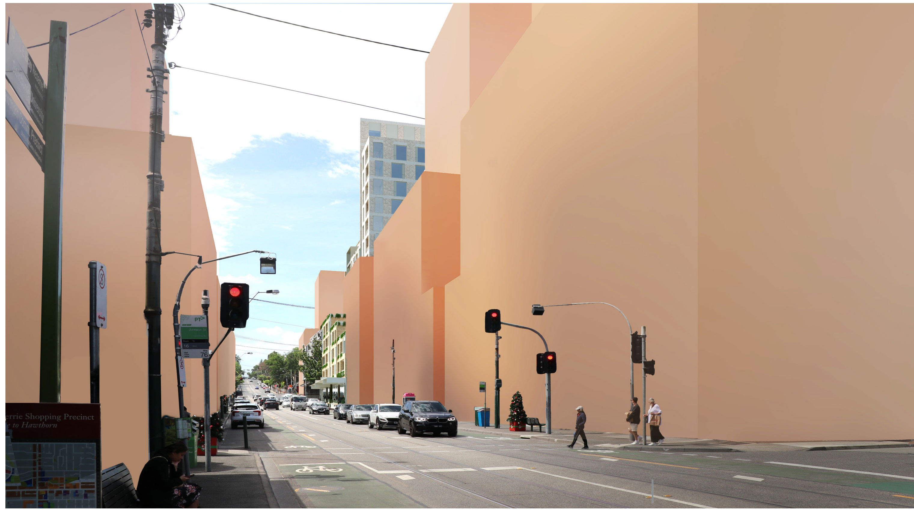
LOOKING NORTH DOWN GLENFERRIE ROAD
