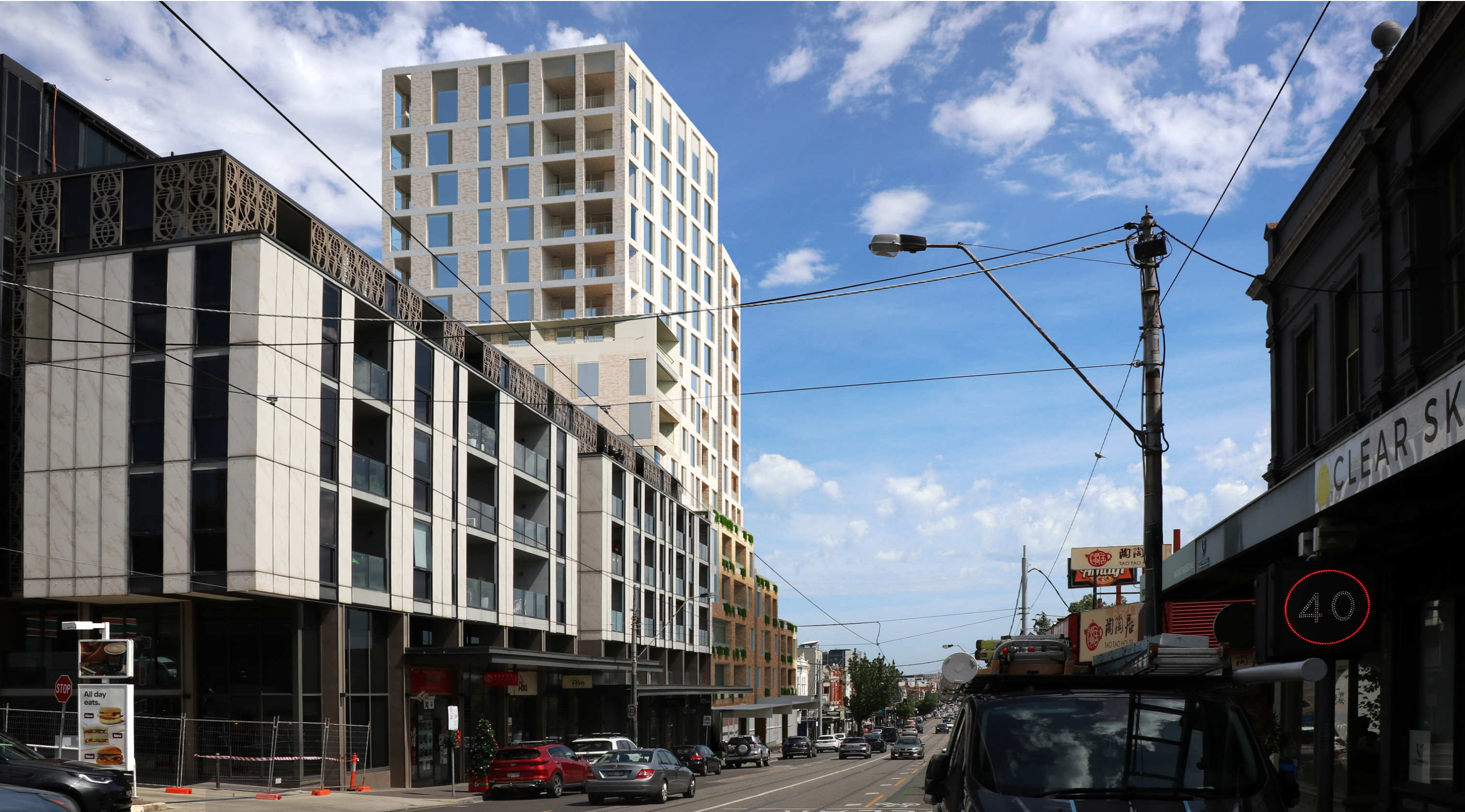
LOOKING SOUTH DOWN GLENFERRIE ROAD
