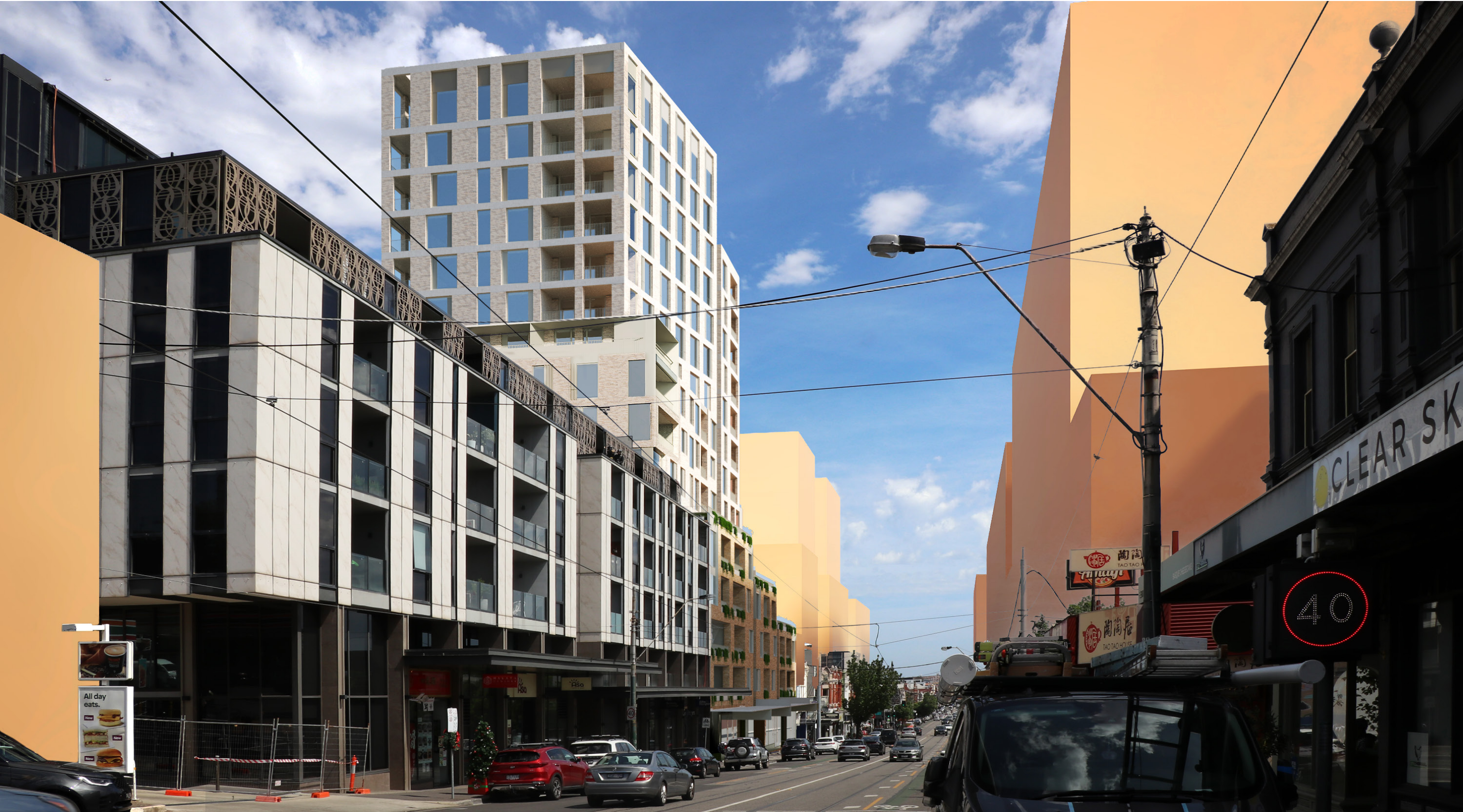
LOOKING SOUTH DOWN GLENFERRIE ROAD
