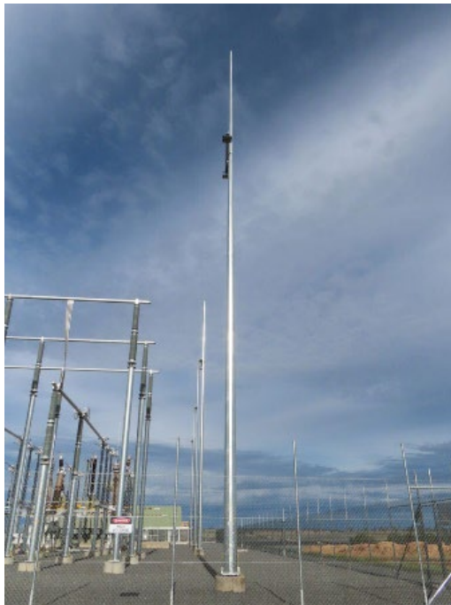
Figure 5 Photo of lightning mast
