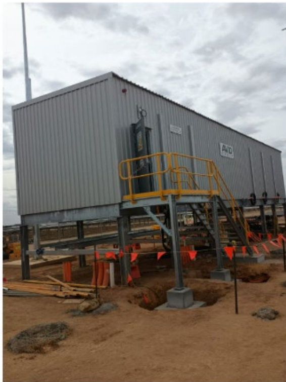
Figure 8 Photo of Raised Demountable Building
