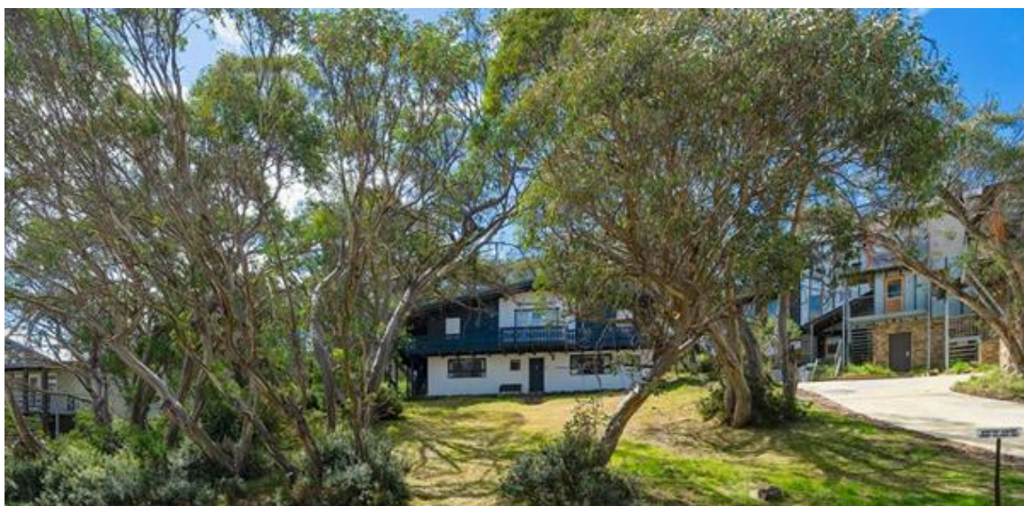
Figure 9 – Photograph of subject site's frontage to Chamois Road – (Source: Application)
