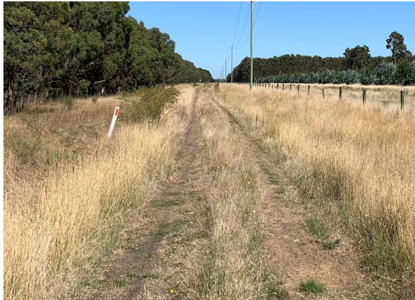
Existing road base
