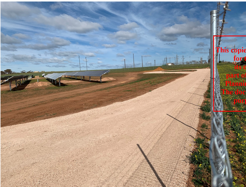
Fig 20. Example road base material that will be used for the solar farm access and tracks (source: Mannum Solar farm)
