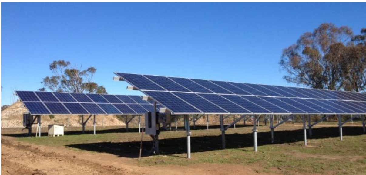
Fig 1. Example Solar PV Array – screw mounted
