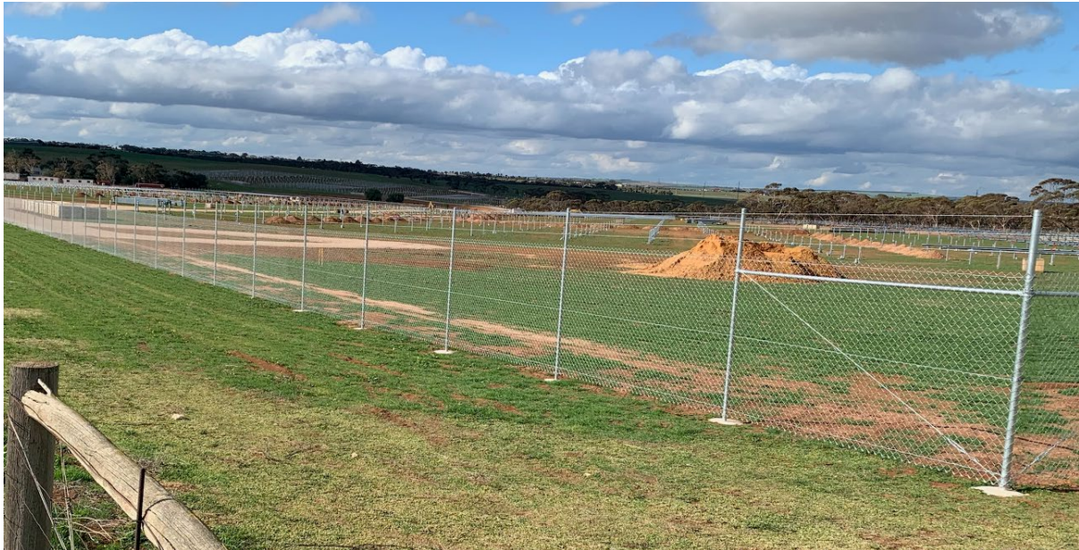
Fig 21. Typical solar farm perimeter fence (Approx. 2.3m high) source: Tetris Energy, Mannum Solar Farm
