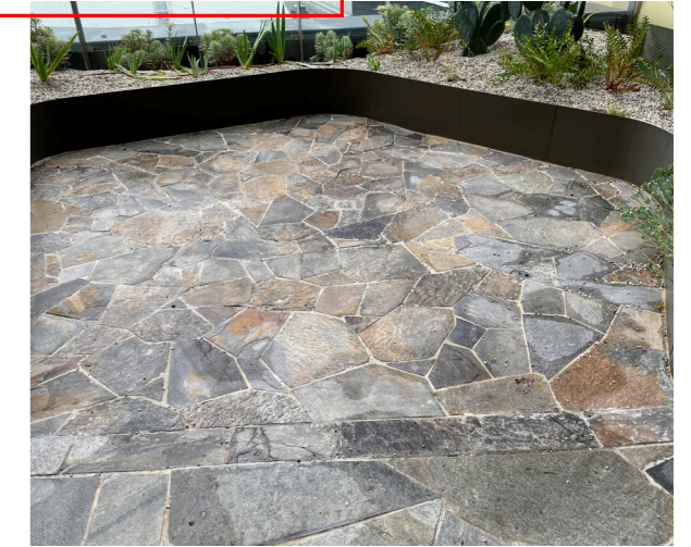
Feature Stone Paving
