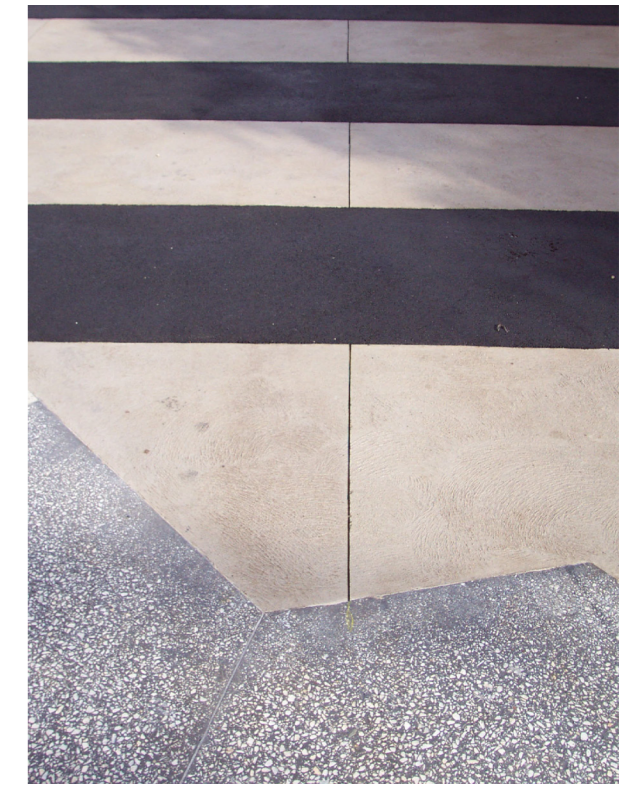
Colour Insitu Concrete & Asphalt Bands
