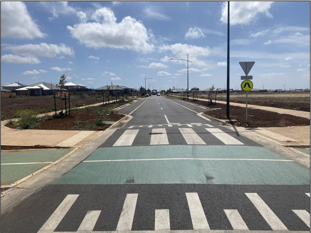
Figure 5 Fuchsia Drive, looking west from adjacent to the subject site
