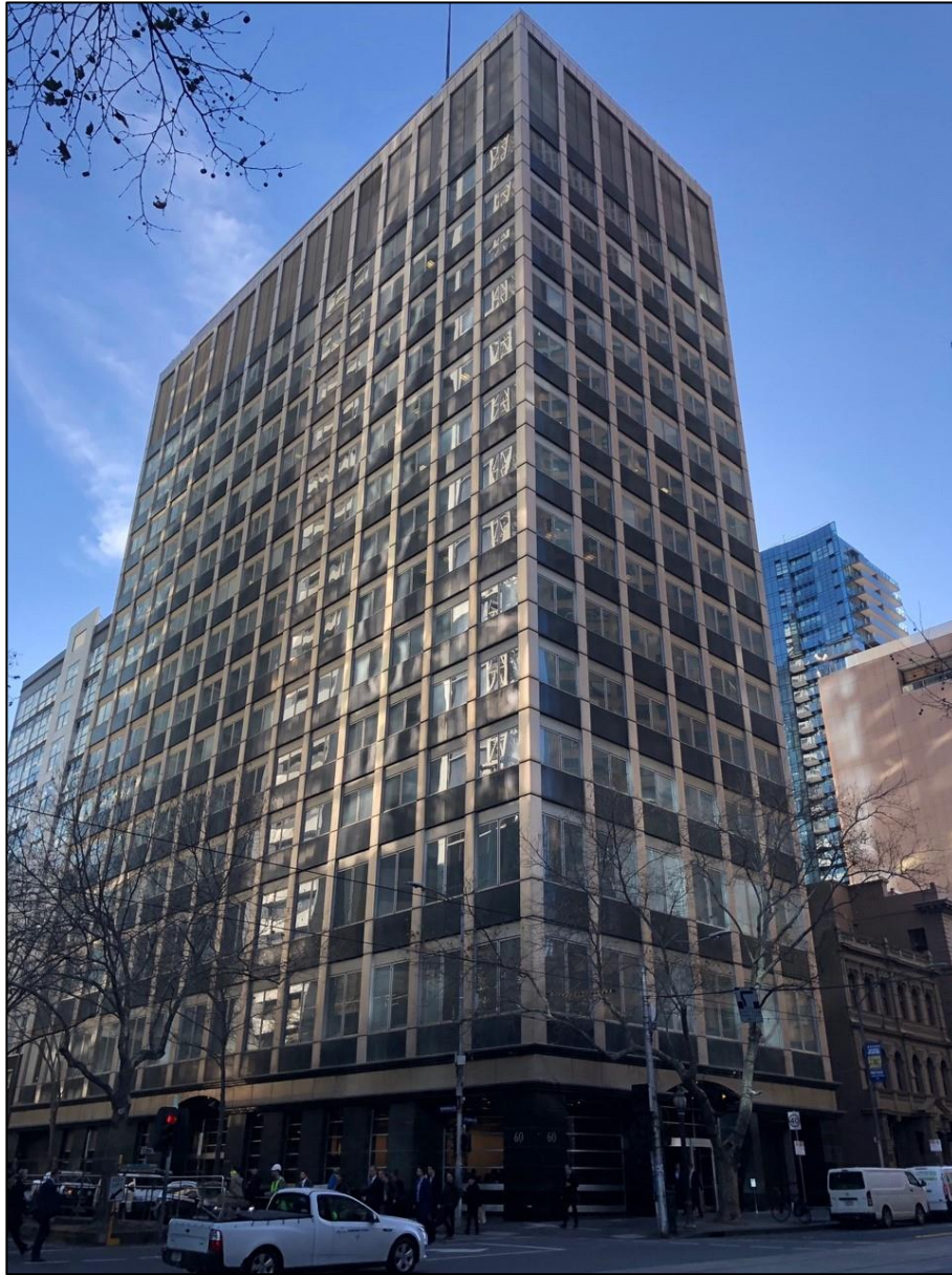
Figure 8 The former RBA building at 60 Collins Street. The original pale marble of the ground floor columns that rose as a continuous vertical expression of structure through the height of the building has been replaced or overclad with segmented steel cladding that is expressly articulated in terms of individual panels. A cornice at the summit of the building replaces the original spandrel panels and further changes the language of the building. At the ground floor, another cornice treatment establishes a visual break between the ground and first floors
