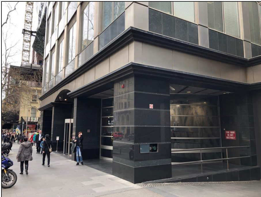
Figure 10 The non-original wide piers, cornices and curved glazed wall to Collins Street.
