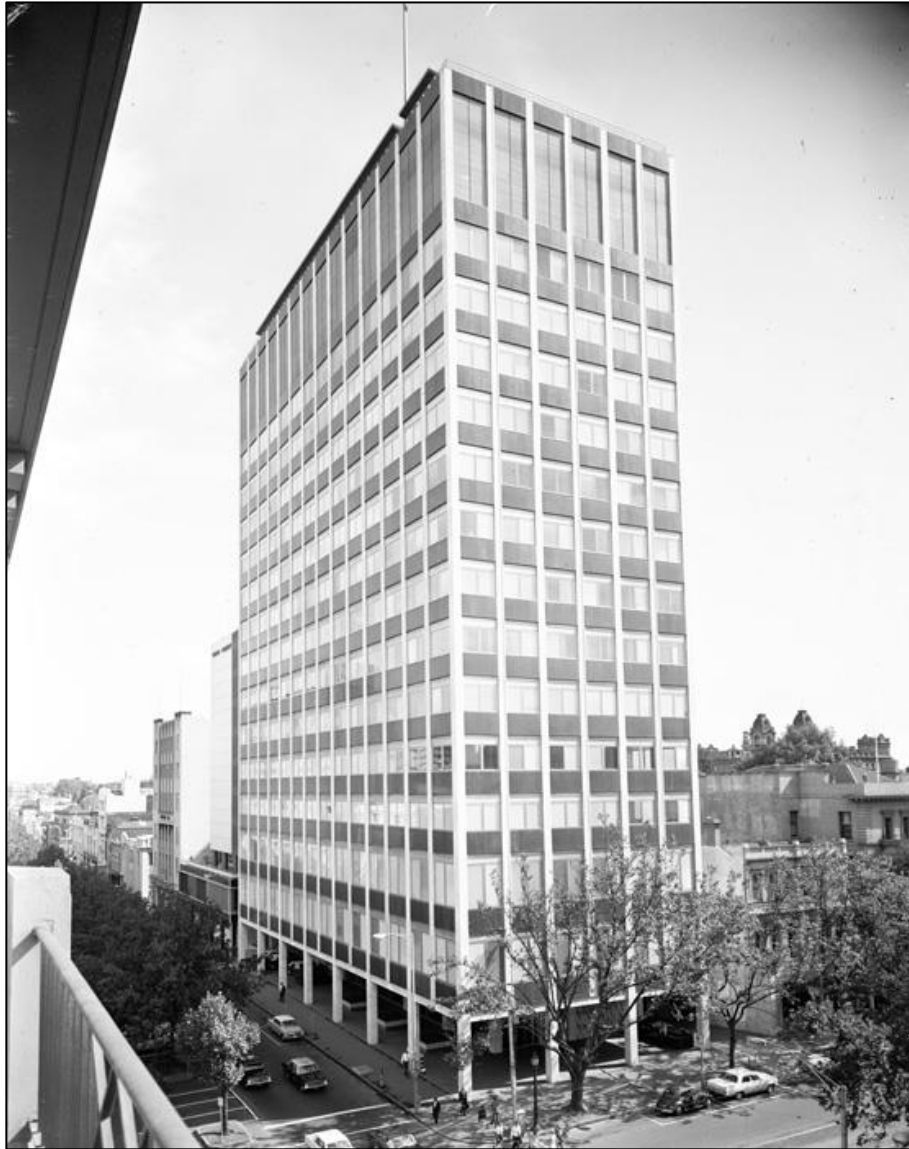
Figure 6 The Reserve Bank of Australia in 1969. Note the pale marble cladding to vertical structural elements including the columns of the ground floor, and the dark granite to spandrels. Note also the recessed ground floor.
