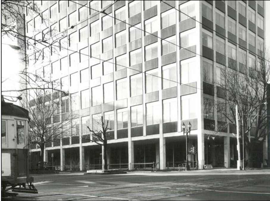
Figure 15 Image showing the lower levels of the building, including the perimeter columns and undercroft concourse to the ground floor in July 1966. Source: Reserve Bank of Australia Archive.
