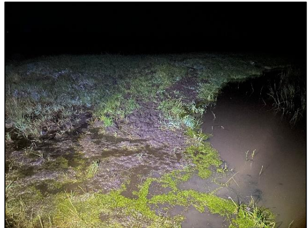
Plate 5. Evidence of plugging from cattle movement around dam 1 (Ecology and Heritage Partners Pty Ltd 08/11/2022).
