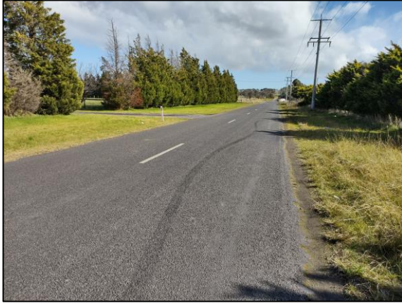
Figure 4: Western Section of Summerhill Rd - View West
