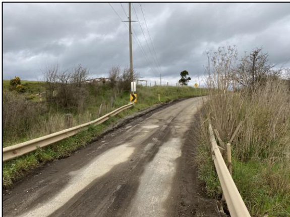
Figure 6: Merri Creek Bridge – View East
