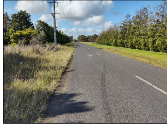
Figure 5: Western Section of Summerhill Rd - View East
