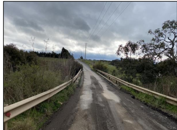
Figure 7: Merri Creek Bridge – View West
