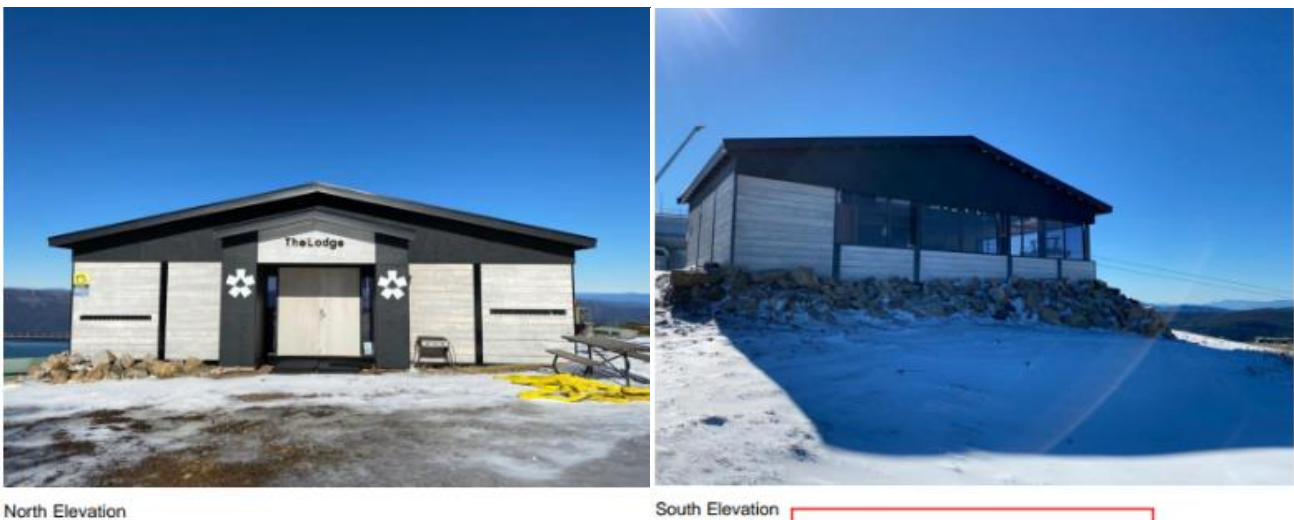
Figure 1: Existing conditions of building, includes the rocks to be removed (Source: Application)
