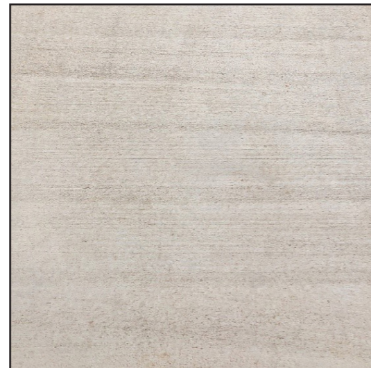
Plain Broom Finished Concrete
