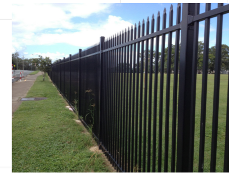
2.4m High Palisade security fence
