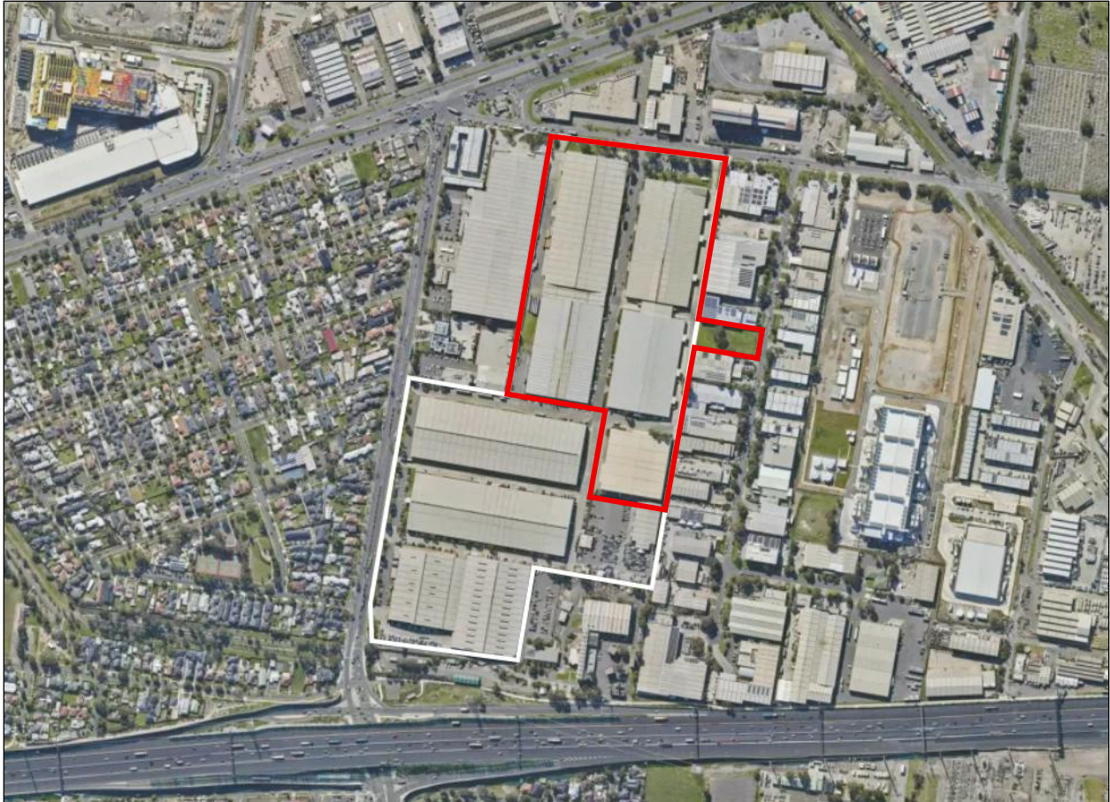
Figure 5 | Aerial Image of the Subject Site (planning unit outlined in red)
