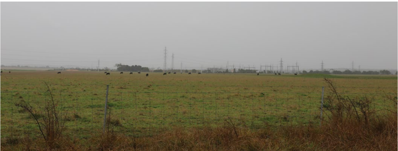
Picture 2 Elaine Terminal Station and associated infrastructure from Elaine-Blue Bridge Road (facing west)
