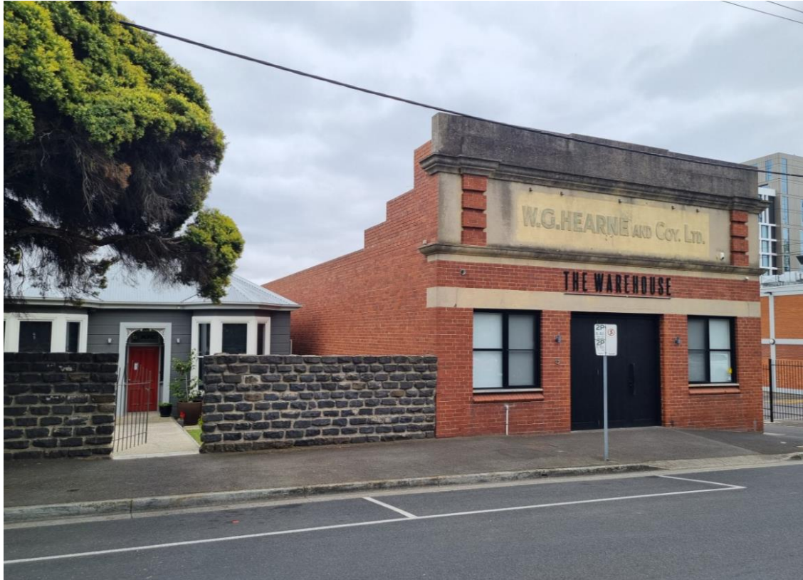
Figure 12: Existing buildings occupying 5 Little Ryrie Street and 12 Wesley Street, Geelong
