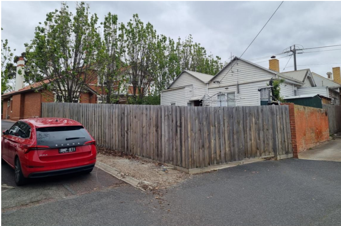
Figure 14: Existing building occupying 257 Princes Highway, Geelong (Viewed from Goodall Lane at the rear)
