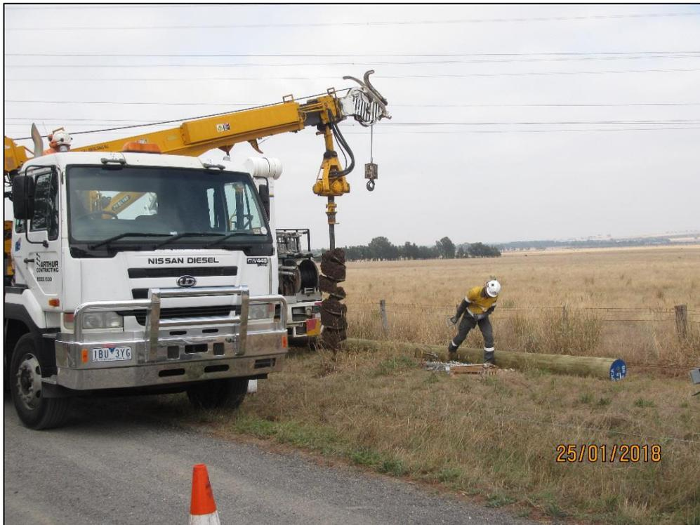
**Photograph 1 – Example of a hole being augured via an arm from truck (note in this example the roadside vegetation was deemed to be non-native, hence the truck parking slightly on the verge and the other truck in the background)**
