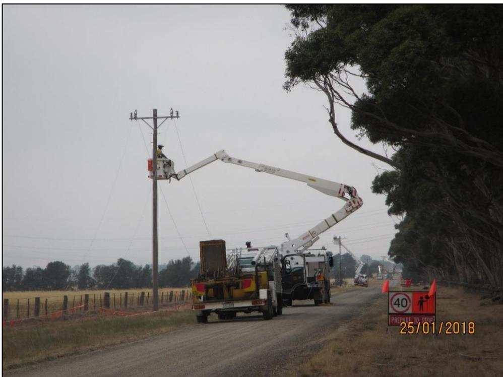
Photograph 4 – Example of contractors working on a new or replacement installation (note the truck is still in the road carriageway)
