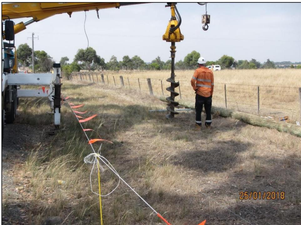
**Photograph 2 – Example of a hole being augured via an arm from truck (note in this example the roadside vegetation was deemed to be native in places and fencing was erected to prevent the truck from entering the road shoulder)**
