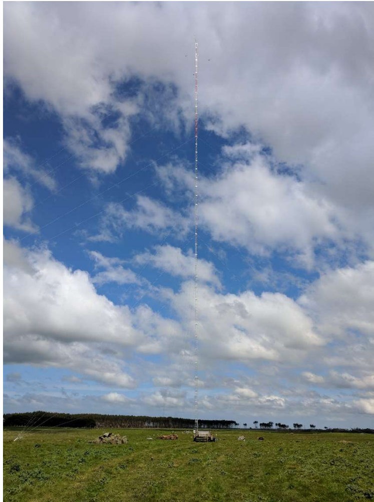
Figure 4: Mast aviation paint and markers
