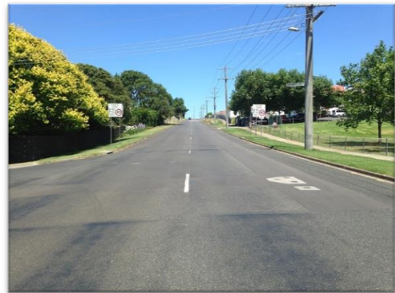
Figure 2.4: Ardlie Street, looking south
