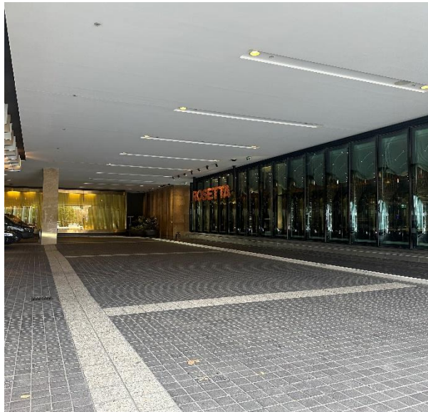
Figure 4: Southern boundary of the existing tenancy showing the Crown Porte cochere (Source: DTP Officer, 2024)
